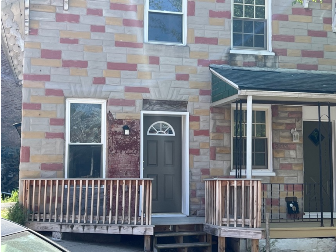
Fig. 33, Formstone Clad Duplex on Buena Vista Ave. with Area of Exposed Brick (source: author's work)
