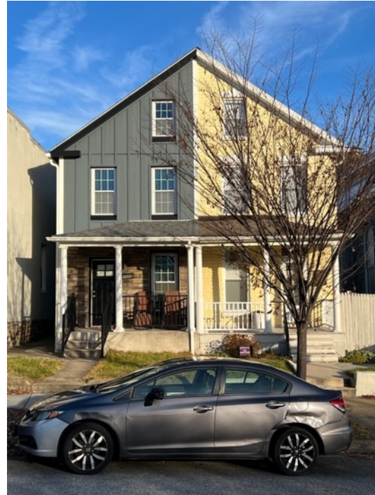
Figure 32b, Duplex on Falls Road, 2022, (source: author's work); Formstone removed from the left side of the duplex, being replaced with modern cladding materials
