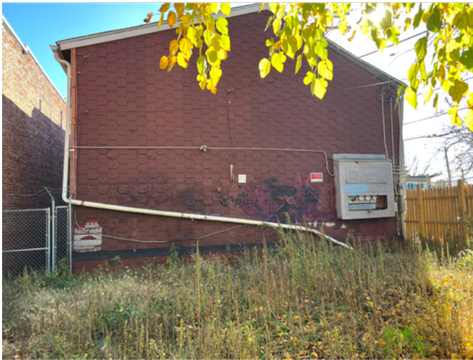
Fig. 19, Rear of building, November 2022 (photo by author)
