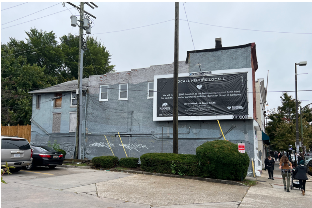
Fig. 17, 1114 W. 36th Street, Western Elevation, October 2022 (photo by author)
