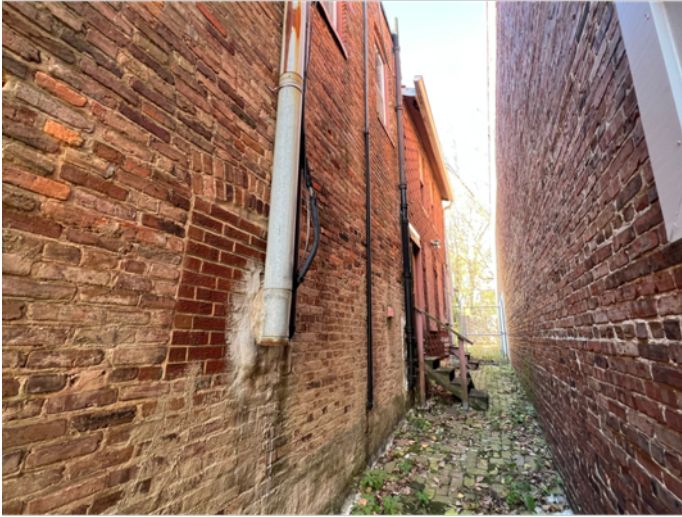
Fig. 18, East side of the building, looking north, November 2022 (photo by Author)
