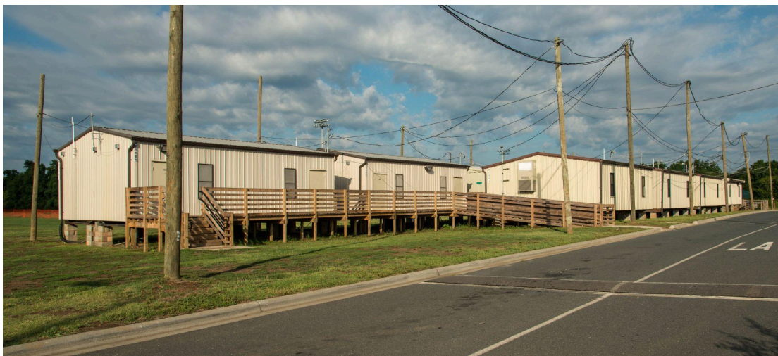
Fig. 1.1: An arrangement of portable classrooms (source: Adobe Stock)
