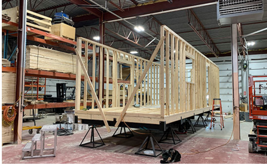
Fig. 2.25: A portable classroom module being built in a factory (source: Boxx Modular)
