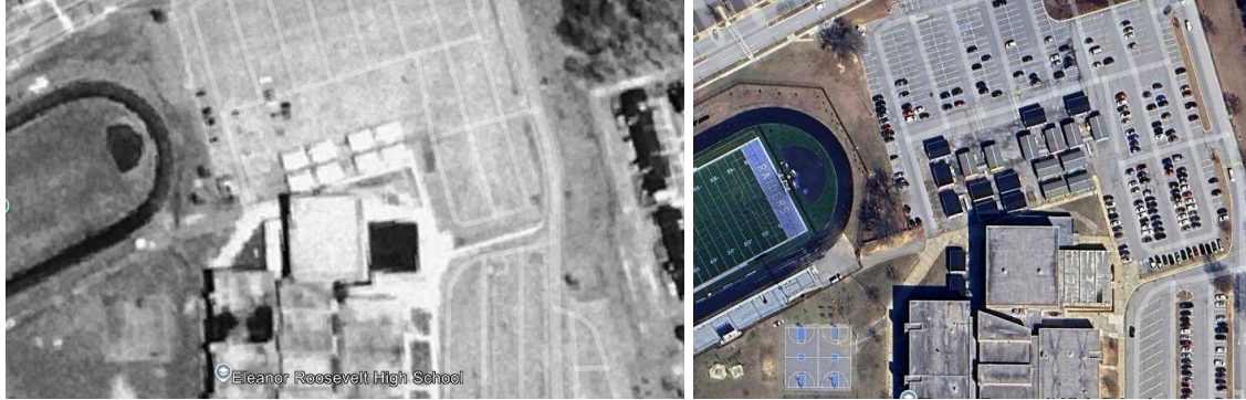
Fig 2.6: The same portables at Eleanor Roosevelt High School (MD) from 1993-2025 (source: Google Earth)
