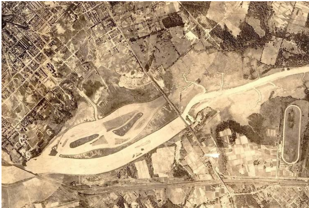
Figure 2- Aerial of progress on dredging the Anacostia River's mudflats to create Kingman Island and Kingman Lake. Note that construction stopped at Benning Rd NE. in this image (1922). Credit: KingmanIsland.com
