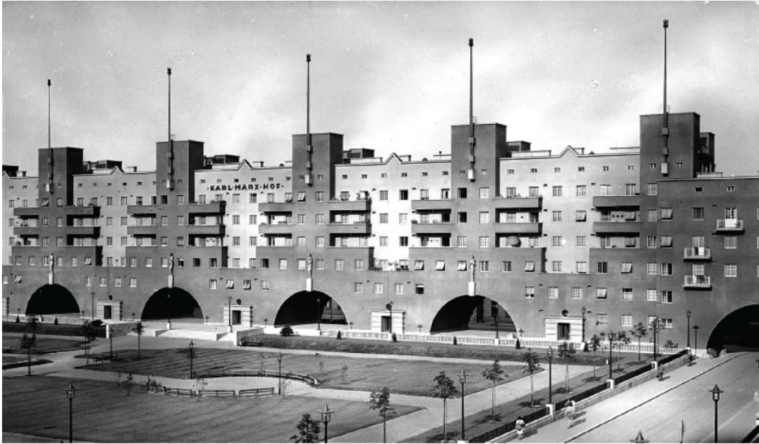
Figure 4.1 Karl Marx Hof façade perspective (source: Hidden Architecture)
