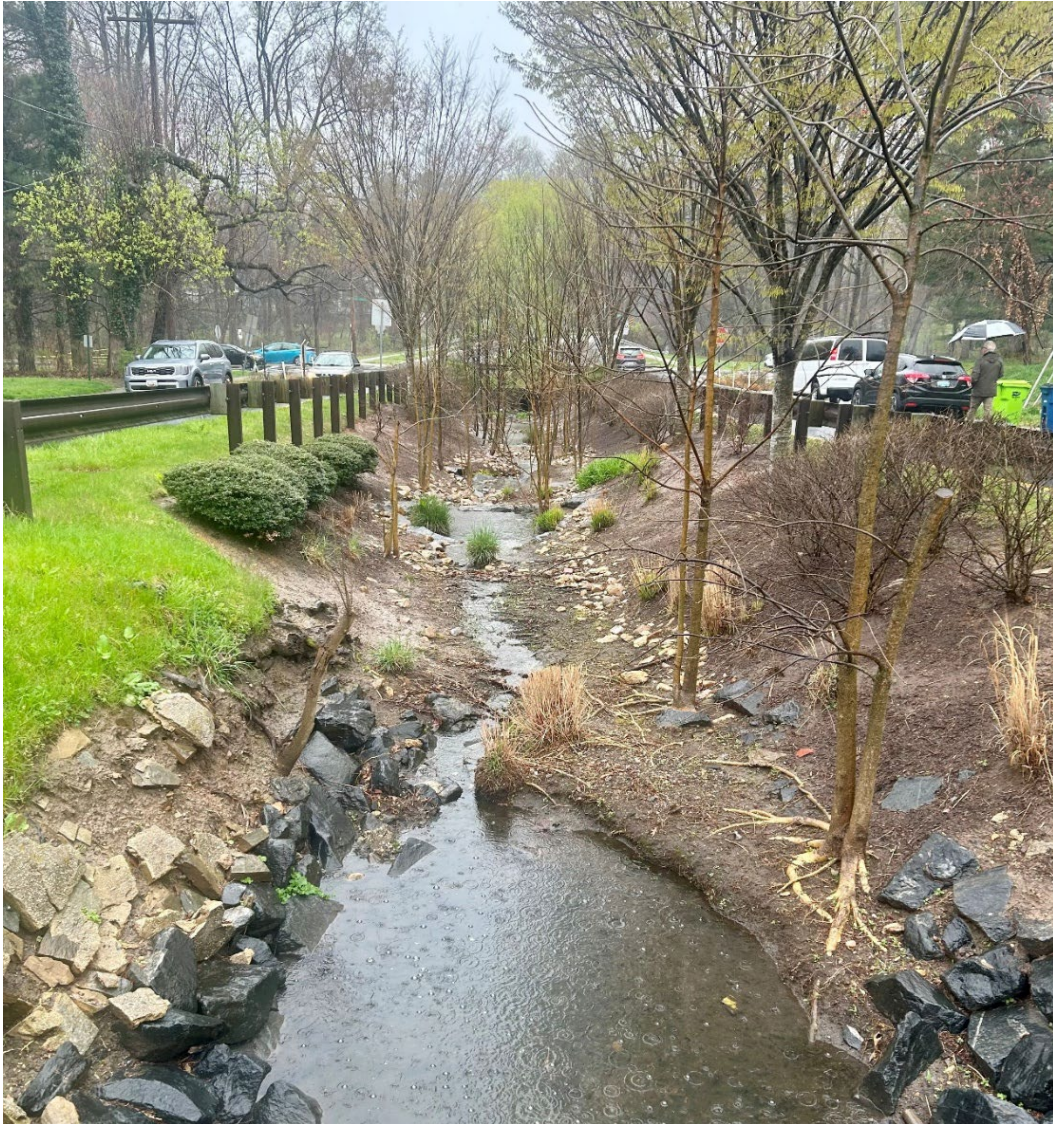
Figure 3.10: Dennis Avenue stormwater intervention, activated. Photo by author
