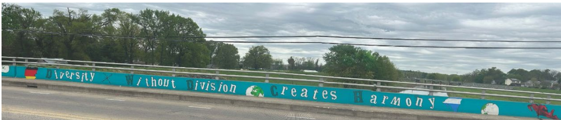
Figure 4.3,4,5: Photos of bridge over NE branch of the Anacostia River, connecting two sides of Edmonston.
