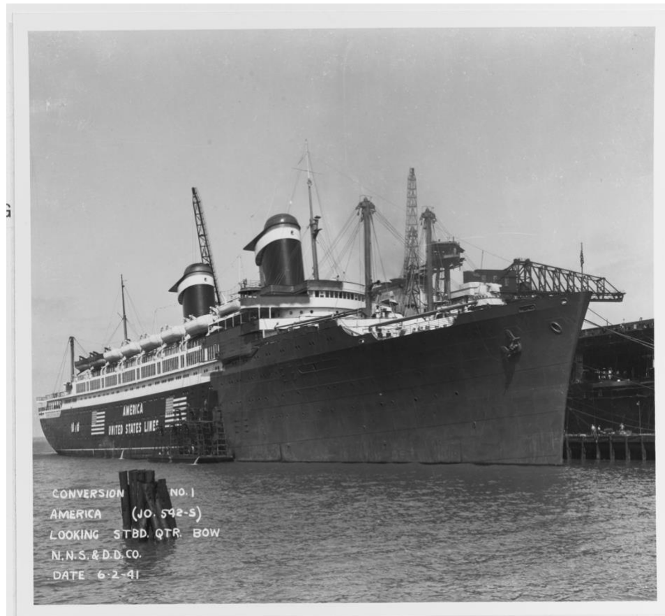
Figure 2: SS America being converted to the USS West Point for service in World War II. Here the ship is halfway through the camouflage paint. (19-N-24561, Archives Branch, Naval History and Heritage Command, Washington, DC)
