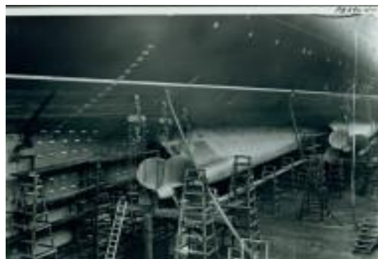
Figure 4: Propeller configuration on the SS United States . Photo Courtesy of the Mariners' Museum.
