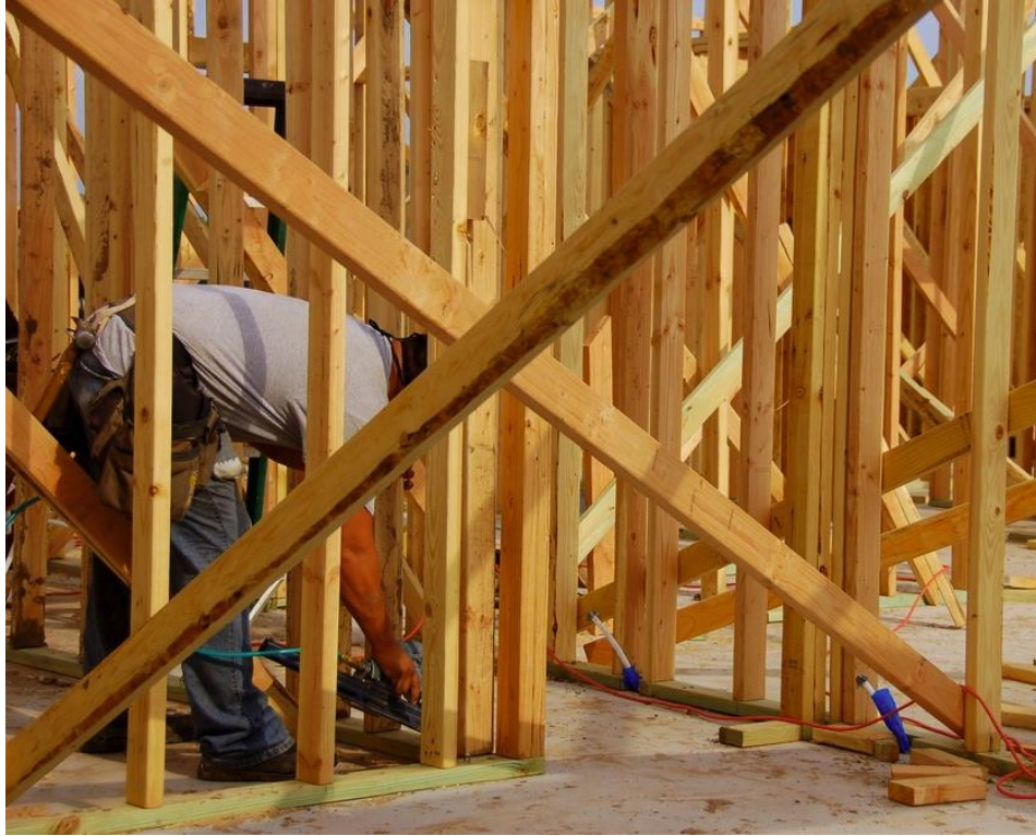
Figure 8: Stick Built Construction. Photograph by Dominick Blocchi, June 07, 2013, Moore, Oklahoma.
