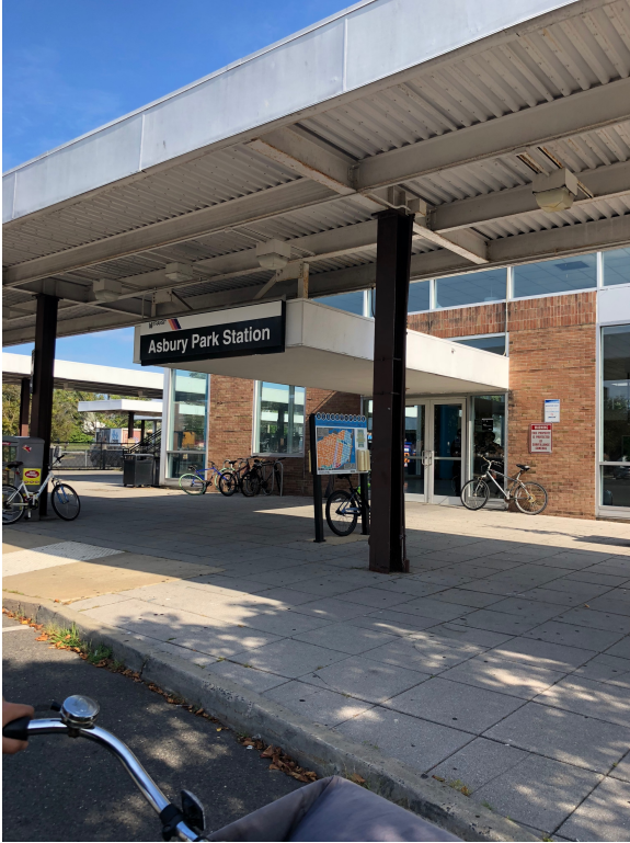
Figure 16 - Asbury Park Station - Source: By Author
