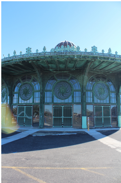
Figure 5 - Carousel Building – Source by Author
