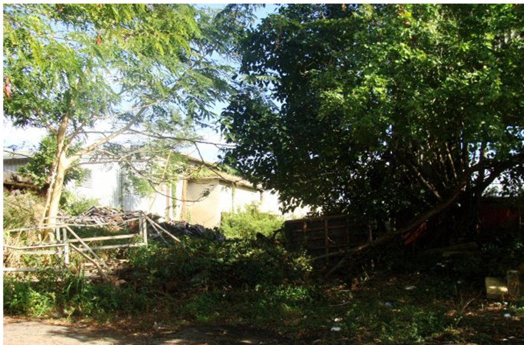
Figure 54: Current Conditions of the Site (Source: Author)
