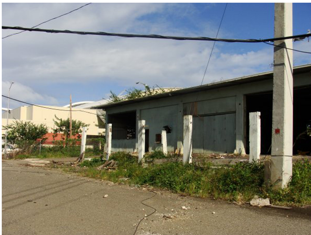
Figure 55: Current Conditions of the Site (Source: Author)
