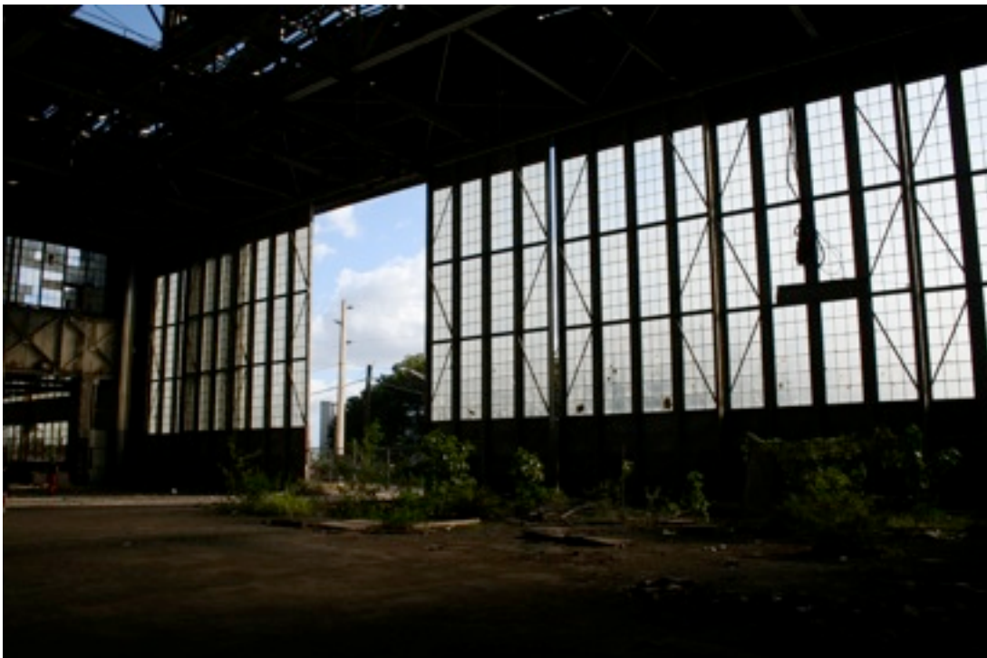
Figure 50: Hangar Doors (Source: Author)
