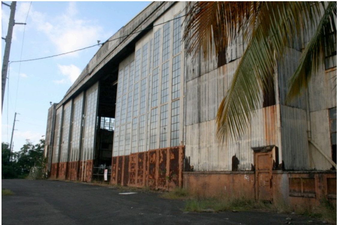
Figure 46: Hangar Exterior (Source: Author)
