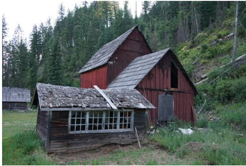
Figure 15: Northeast view of shop, barn, root cellar, and chicken house in foreground. Photograph, courtesy of the author.
