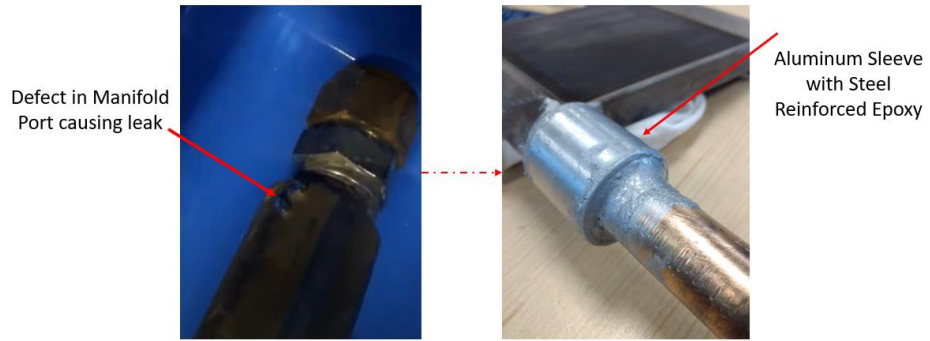
NTHX1 Leak Repairs
