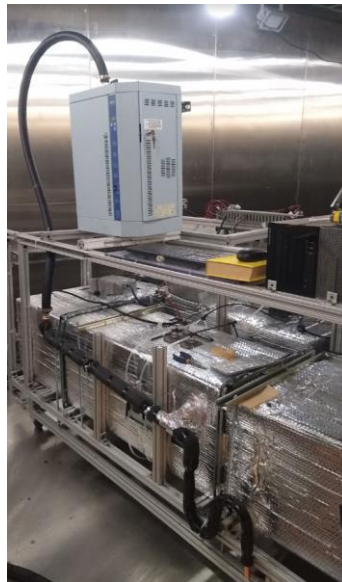
Figure 89: 4kW Steam Humidifier Installed onto Evaporator Loop.
