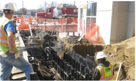
Silva Cell Installation
