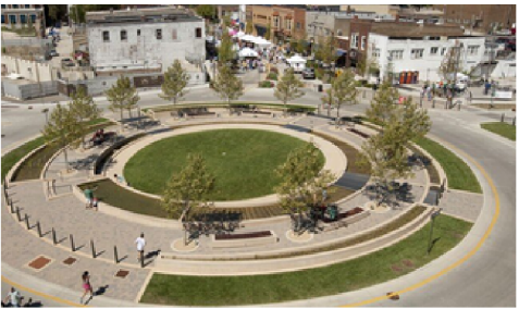
Silva Cell Installation
