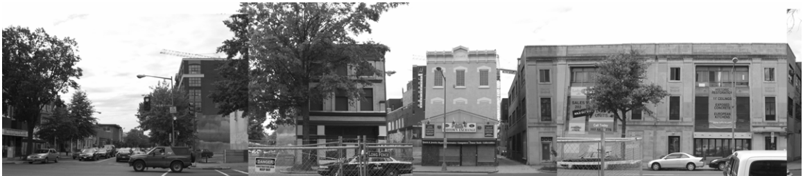
Figure 20: Western Side of 14 th Street
