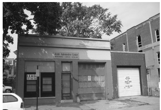
Figure 29: Automobile Repair Shop on Church Street
