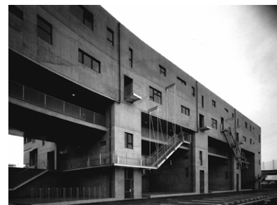
Figure 83: View of North façade [Holl 95]
