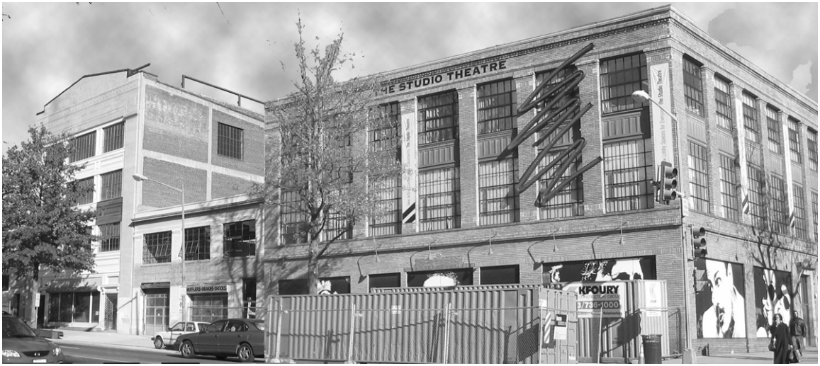
Figure 34: Existing Studio Theater and Two Adjacent Buildings
