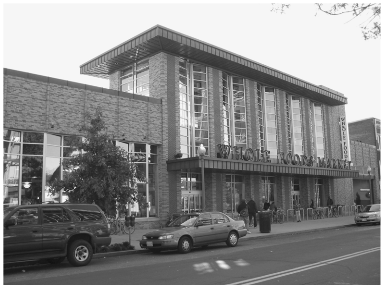
Figure 39: Exterior of Whole Foods Market
