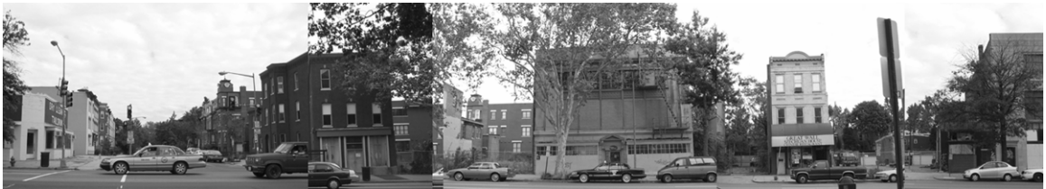
Figure 23: Eastern Side of 14 th Street
