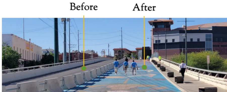
Figure 15: Durango Street Bridge Comparison of Traditional and Painted Asphalt. Source: Cheng & Kaur, 2022.
