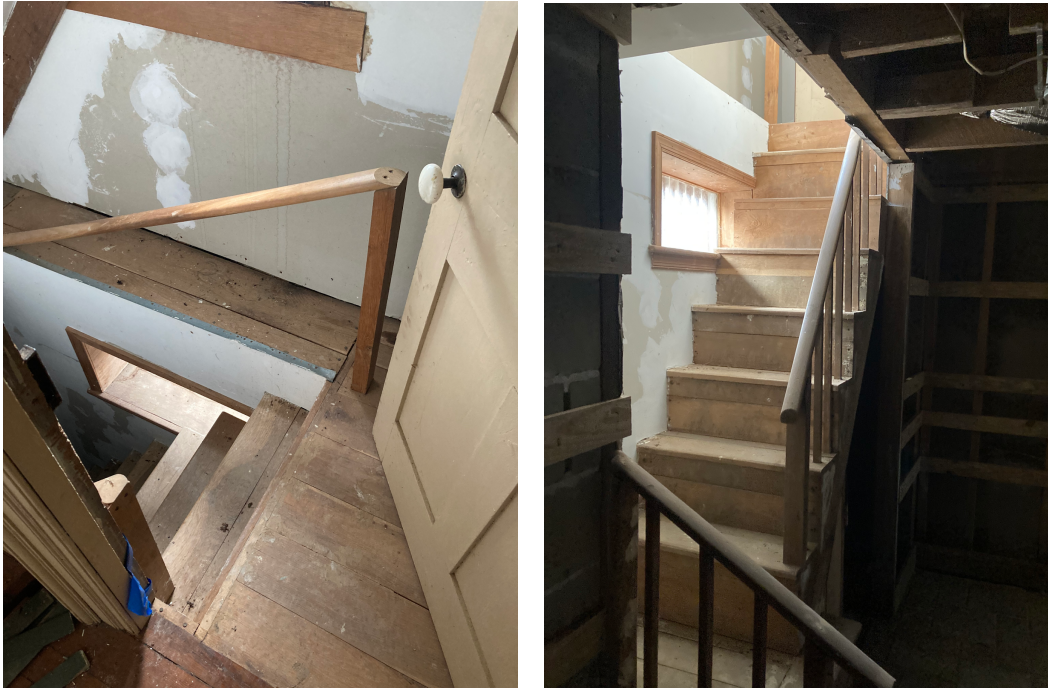
Figure 3.7. (left) Interior entrance to basement. The apron of the first floor window is visible along the top. The small basement window can be seen along the stairs leading into the basement. (right) Interior entrance to basement, view from basement (Photo by author, 2022).
