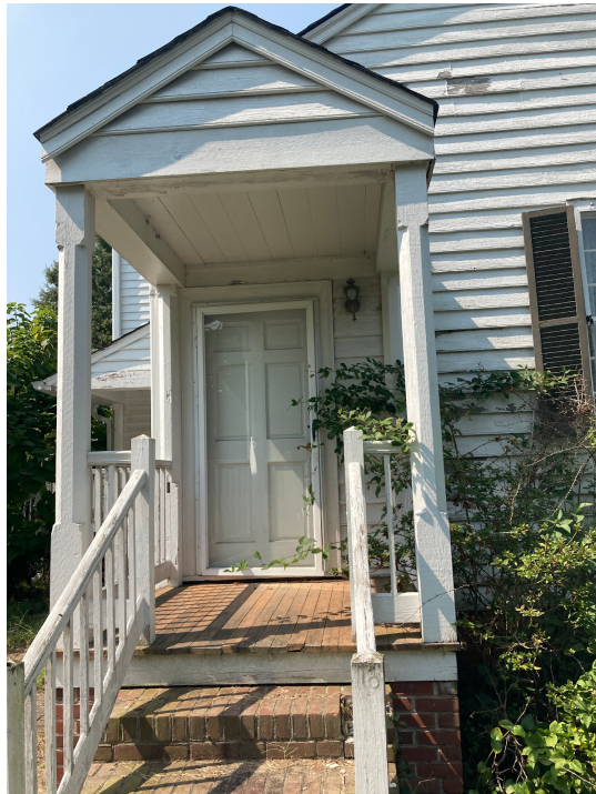
Figure 3.24. Exterior of the servant door outside the dining room (Photo by the author, 2022).
