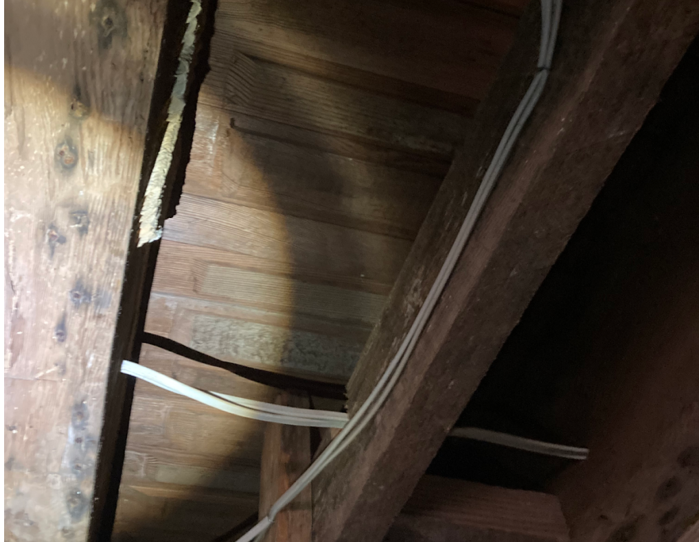
Figure 3.9. Tongue and groove flooring visible between joists (Photo by author, 2022).
