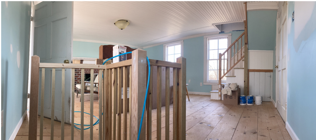
Figure 4.13. Kitchen Remodeling (Photo by author, 2022).
