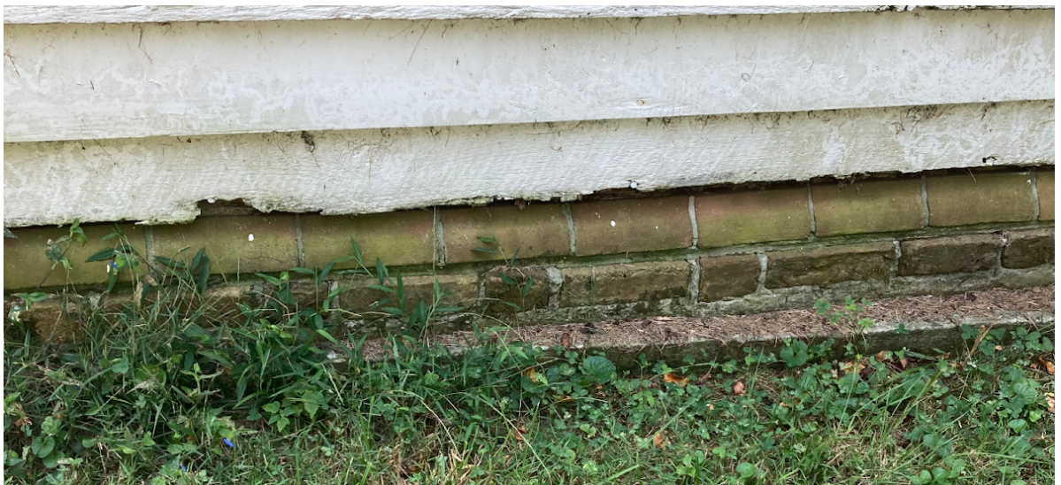
Figure 3.46. Back of storehouse with a concrete slab in the brick foundation (Photo by author, 2022).
