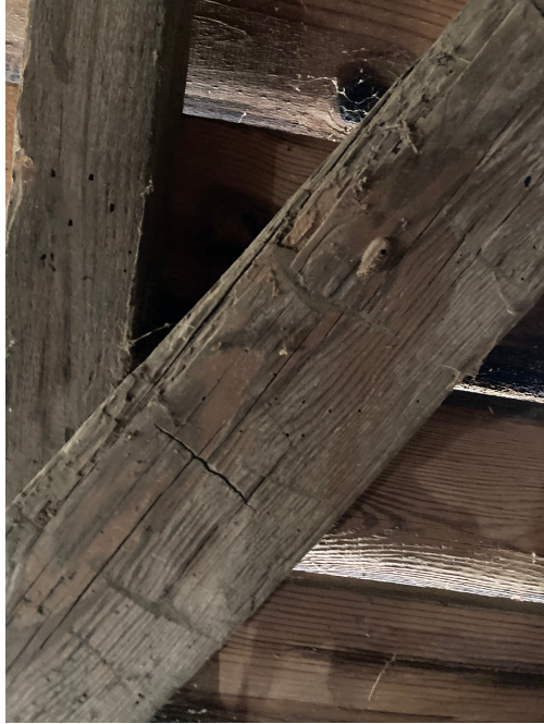
Figure 3.29. (left) Hand-hewn rafter in attic, (right) Pit or sash sawn rafter (Photos by author, 2022).
