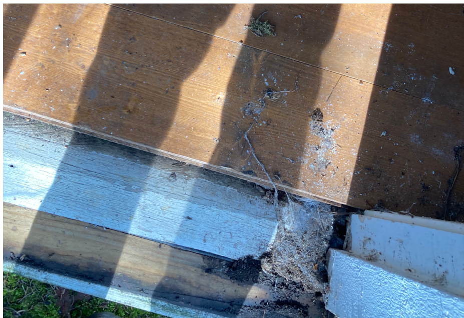
Figure 3.50. Tongue and groove flooring visible on door sill Photo by author.
