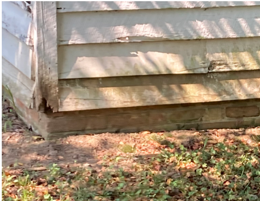
Figure 3.43. Dairy foundation (Photo by author, 2022).
