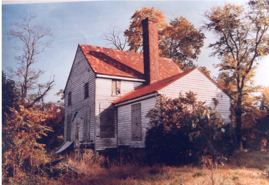
Figure 4.0. The rear of Woodburn, 1970s (Source: Tyler Family Collection).
