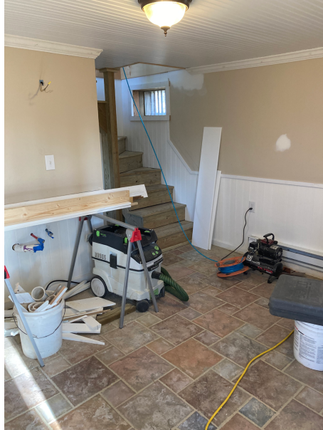
Figure 4.14 - Kitchen basement remodeling (Photo by author,2022).
