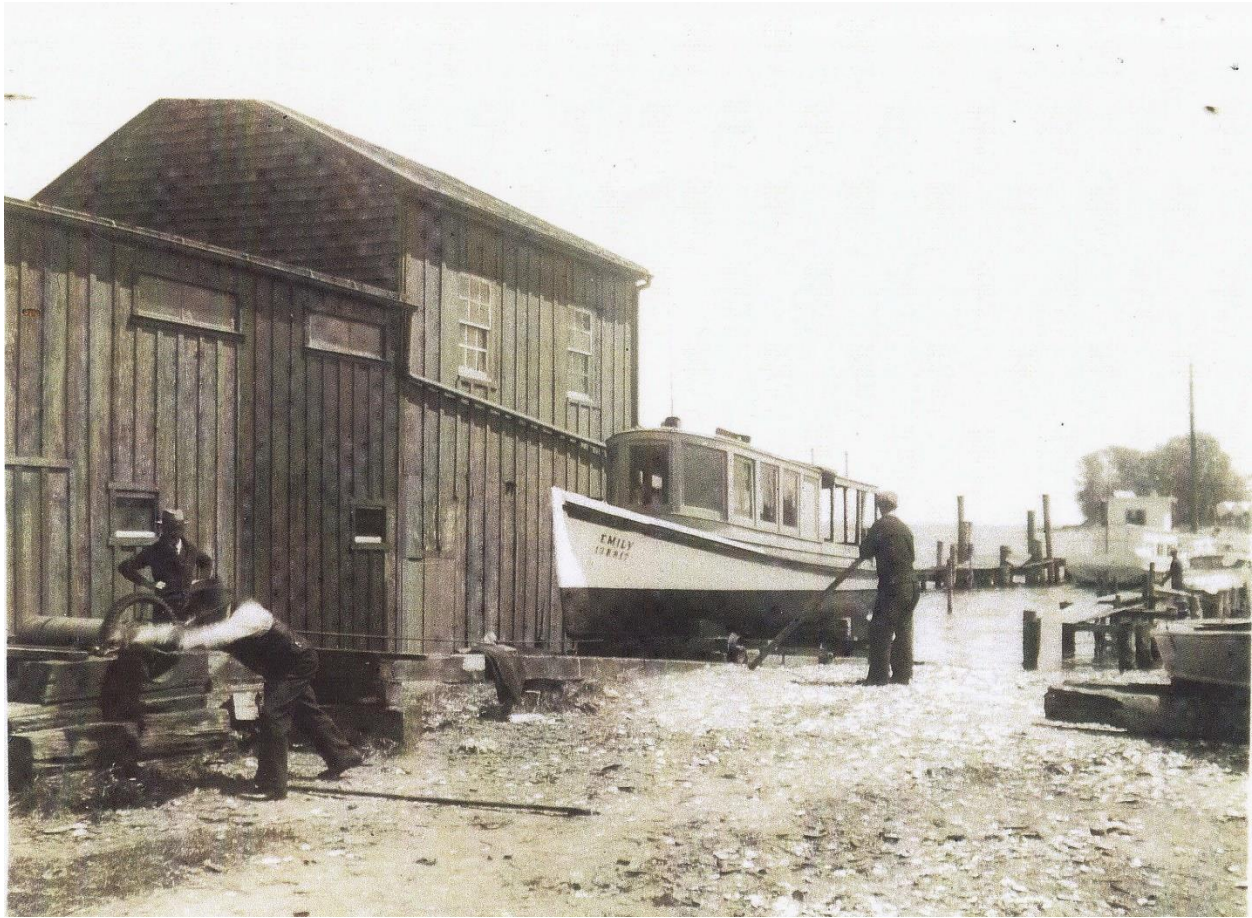
Figure 5. Rear of the boat shed and landing shed showing manual operation of a marine railway. Image likely from 1920s – 1930s. Source: Burtis Family
