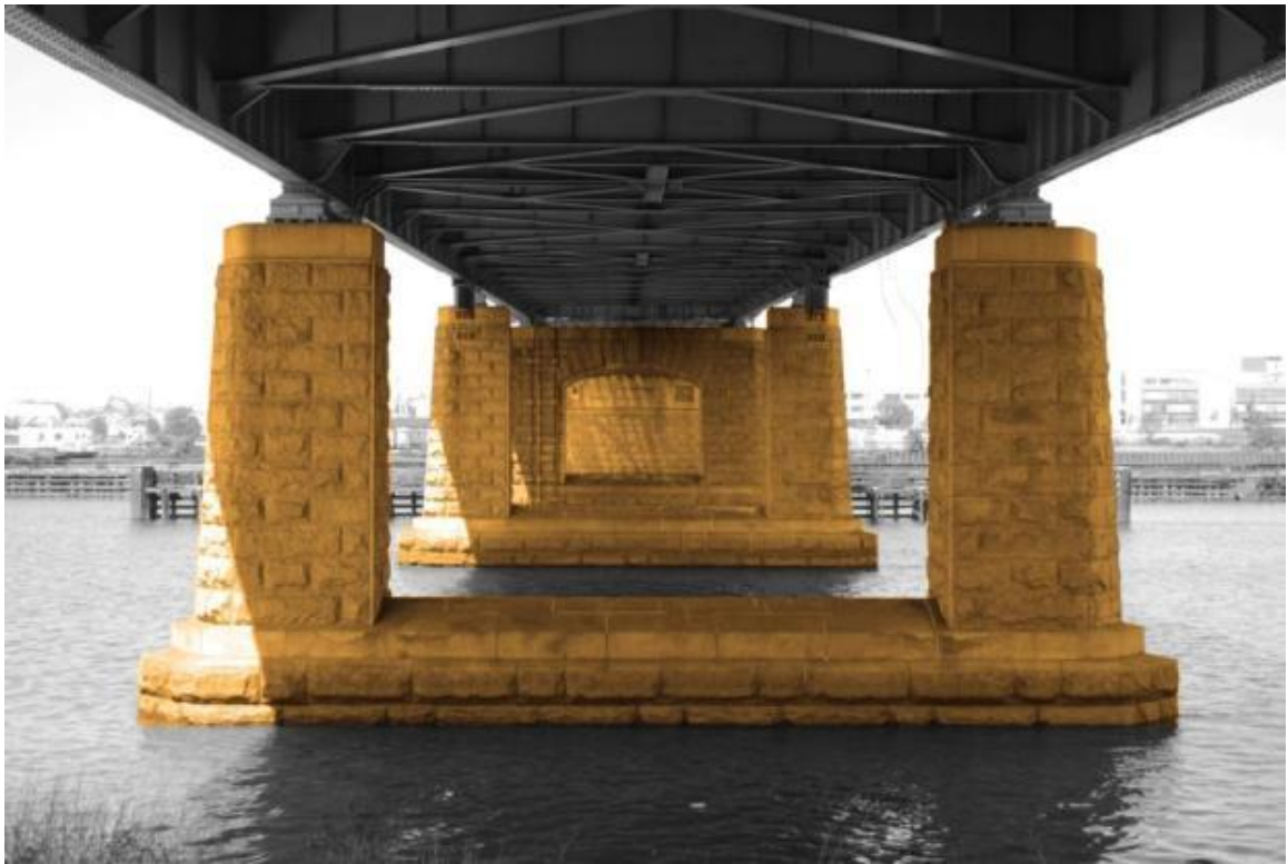
Figure 18: Masonry Support Piers [Aroom]
