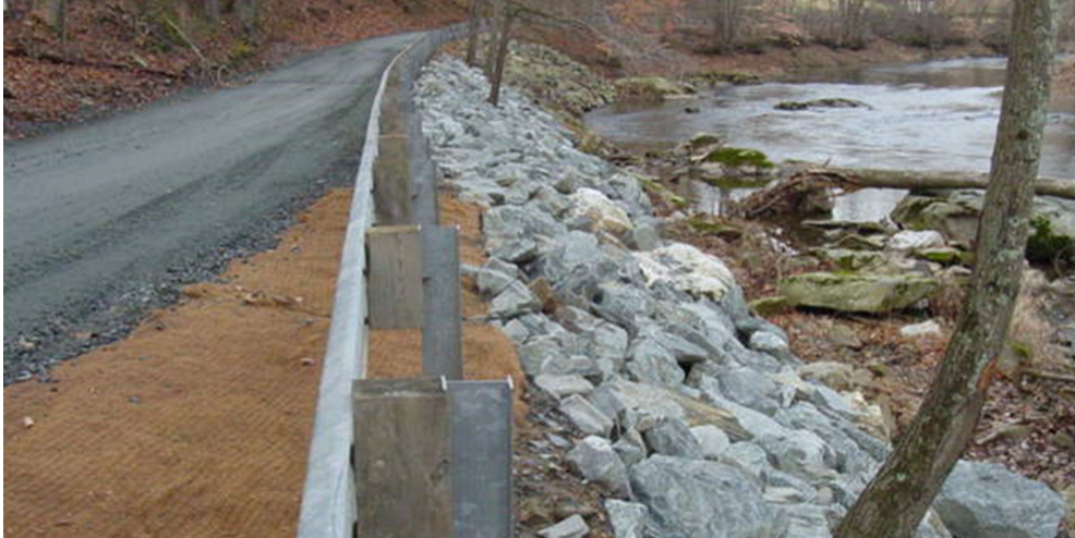
Figure 2. Repaired road embankment (Jeff Stratmeyer, Harford County Department of Public Works)
