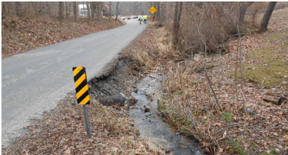
Figure 1. Eroded road embankment (Jeff Stratmeyer, Harford County Department of Public Works)
