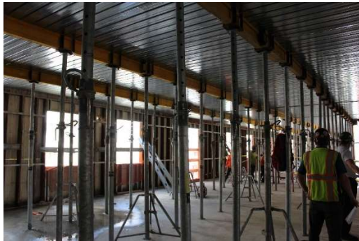
Fig. 5.2 Initial condition of composite slab.
