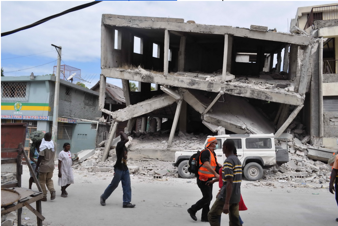
Fig. 3 - Collapse of an unfinished 4 story building after the 2010 earthquake in Haiti. Obtained from: http://eqclearinghouse.org/co/20100112-haiti/general-information/fierro-photos-part Accessed April 2018.
