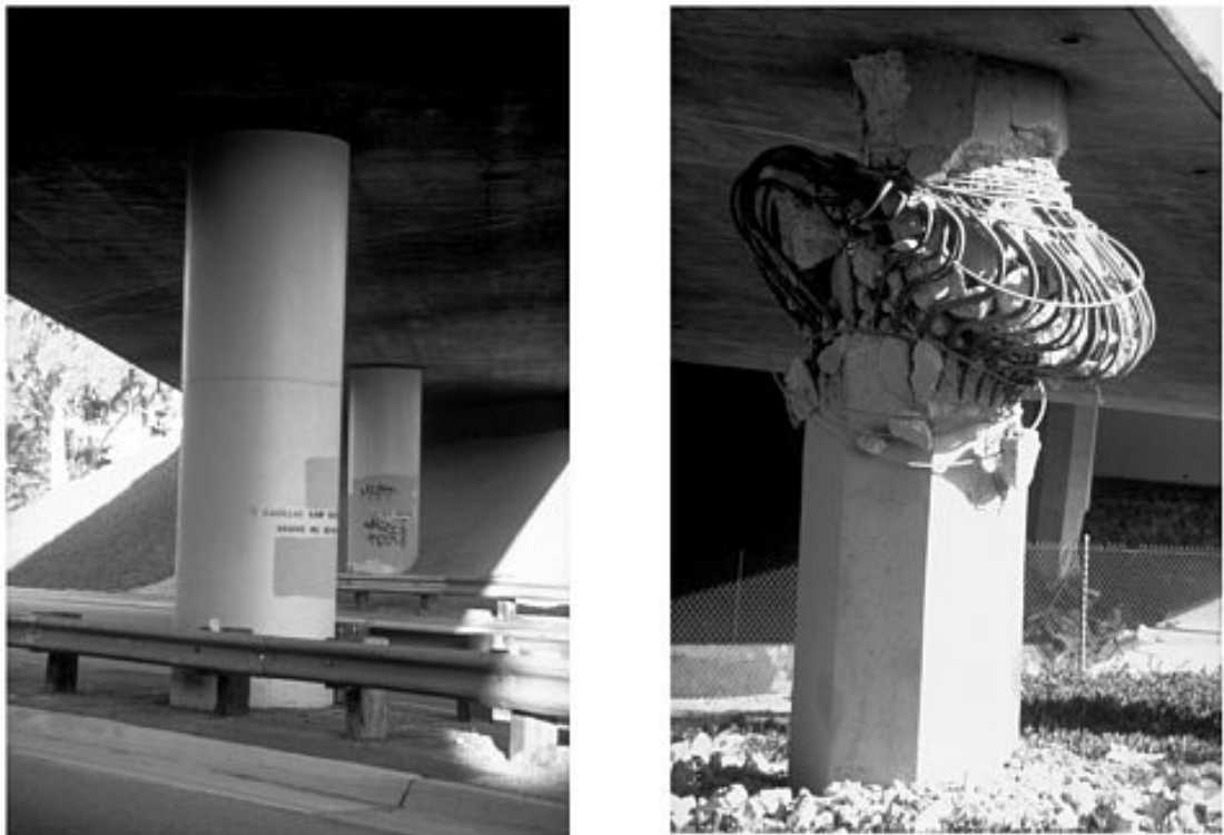
Fig. 6 - Comparison of retrofitted and unimproved concrete bridge columns following the 1994 earthquake in Northridge, California. Obtained from: https://www.nap.edu/read/10799/chapter/3#24 Accessed April 2018.
