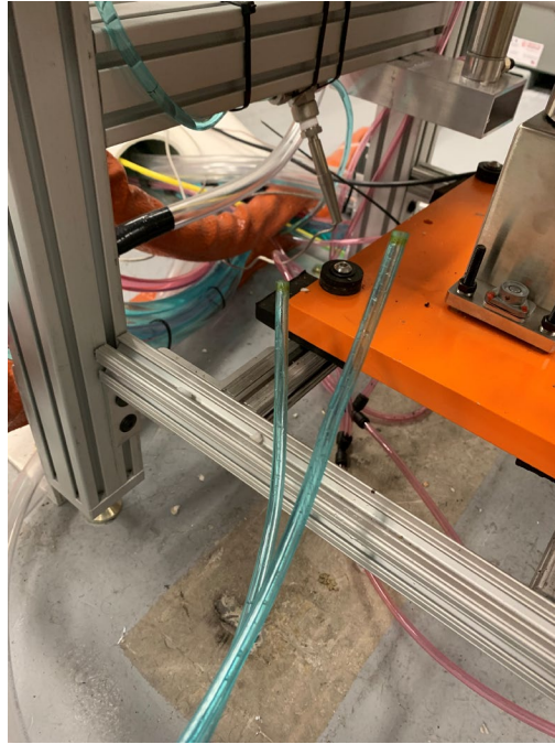
Figure B.15: Open ends of water lines set aside at FPA.
