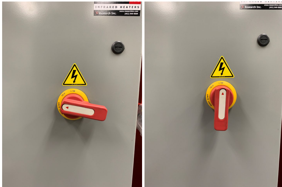
Figure B.6(b): FPA lamp controller power switch turned to the on position.
