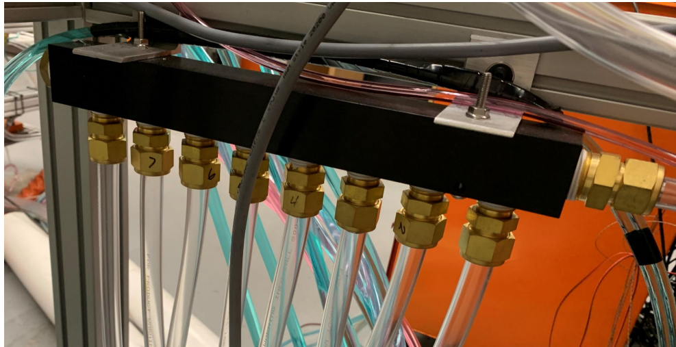
Figure 2.7(a): Upstream distribution manifold.
