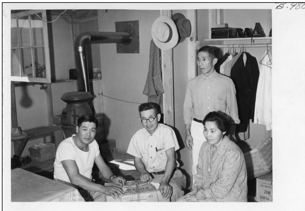
Figure 3-5. Example of the interior of the barracks with a pot-bellied stove. Courtesy of the National Archives, photo no. 210-G-16B-970, Densho Digital Repository
