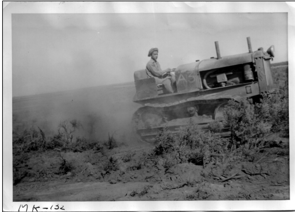
Figure 3-6. “An evacuee drives a heavy tractor pulling a triangle to heavy railroad irons breaking off sagebrush. This is one of the methods of clearing off land of the sagebrush adjacent to the Minidoka Relocation Center.”
