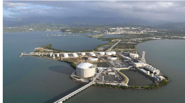
Fig 6.3 EcoElectrica Power Plant (Source: Matrix PDM)
