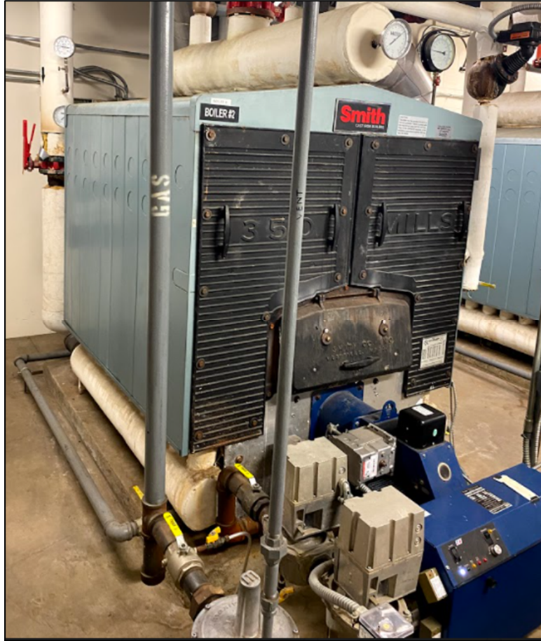
Figure 23: Boiler Serving the Kent McCanner Elementary School Building
