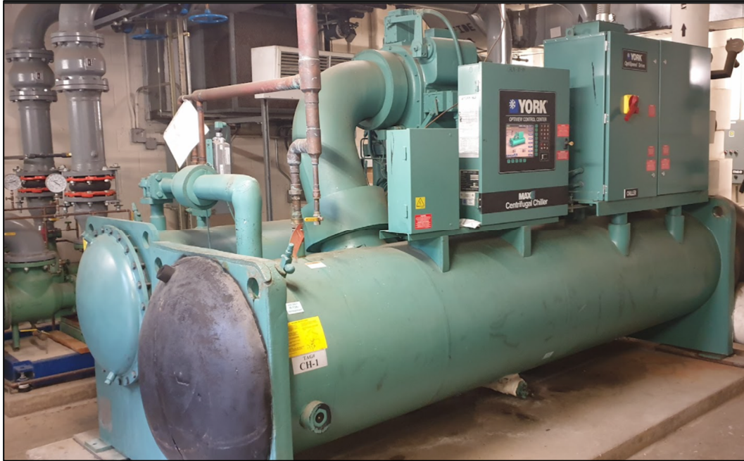
Figure 22: Chiller Serving the Kent McCanner Elementary School Building
