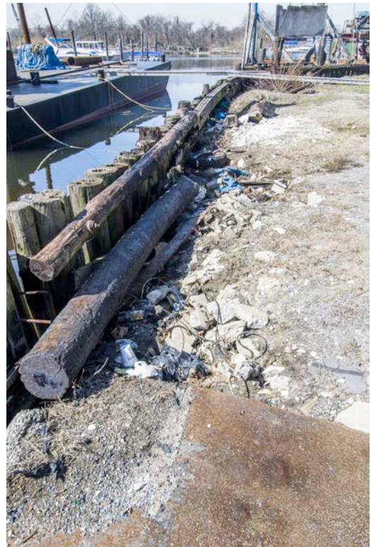
FIGURE 55. Existing Site Shoreline Stabilization on Site (Wierengo)
