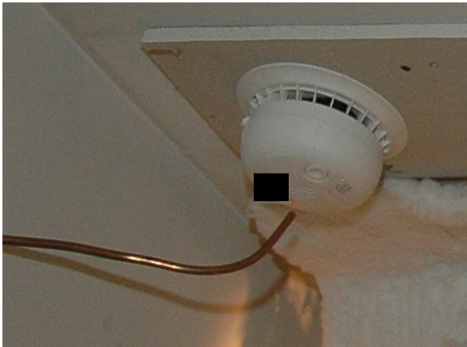
Figure 9-2. Acoustic monitor tubing placement
