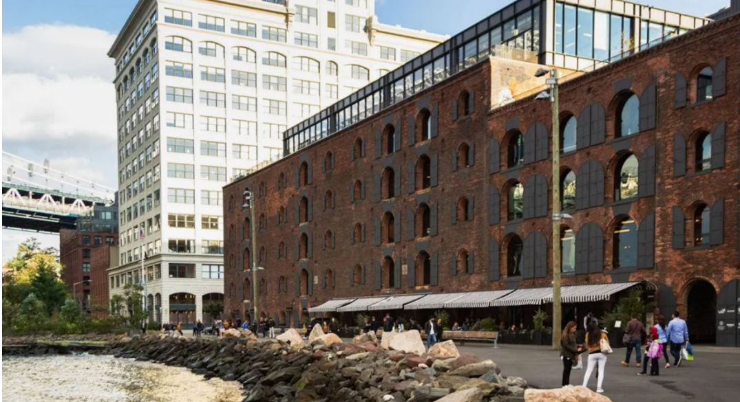
Fig. 9 Empire Stores from the East River, Brooklyn, NY. Image Credit: Empire Stores
