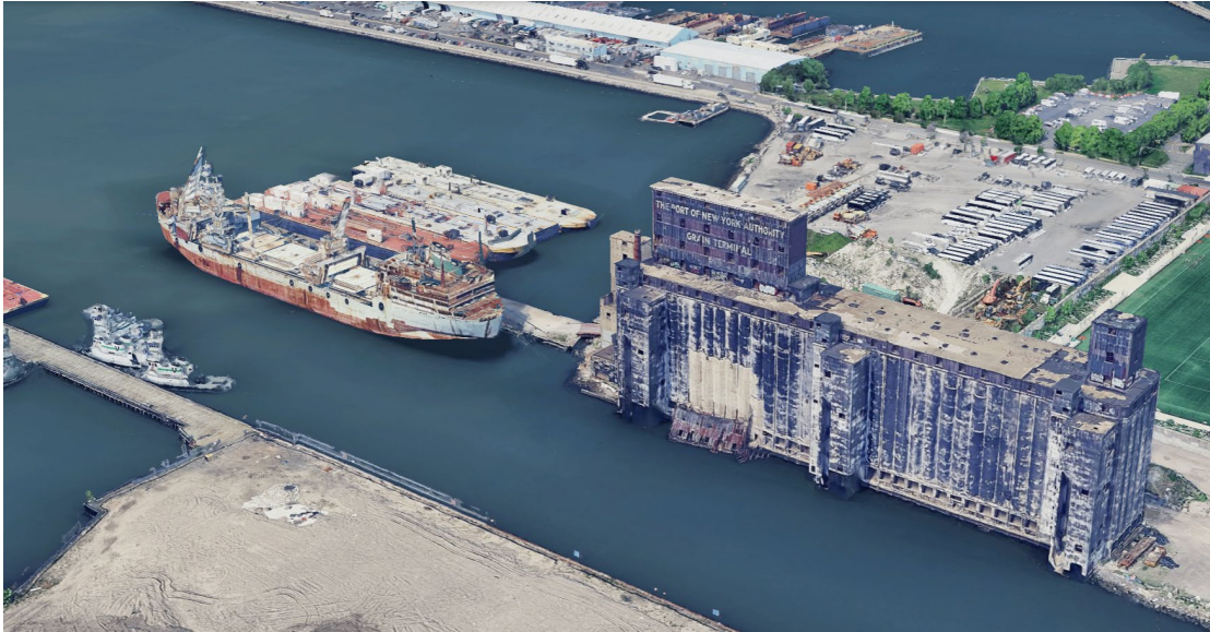
Fig. 40 Red Hook Grain Terminal as it appears in the present. Image Credit: Google Earth.
