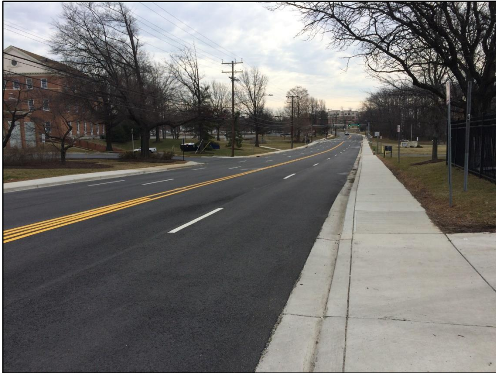
Figure 5.12: Newly Paved Road
