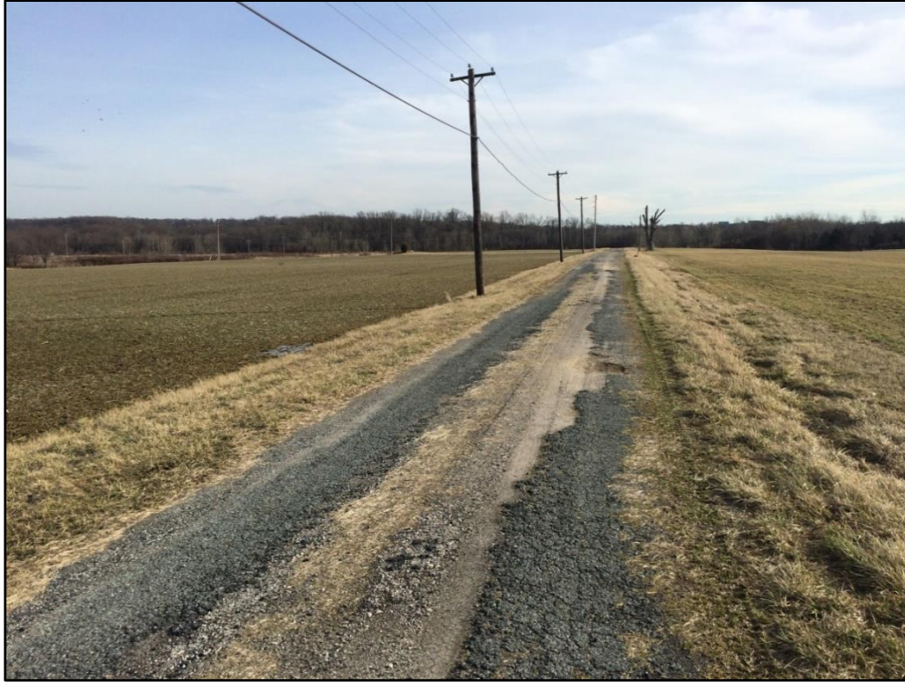
Figure 5.16: Damaged Pavement
