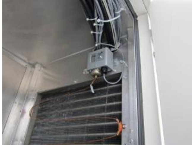
Figure 33: Picture of a generic freeze stat
