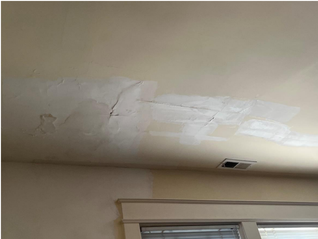
Figure 48. Plaster repair in the living room. Photograph taken by author on January 18, 2023.
