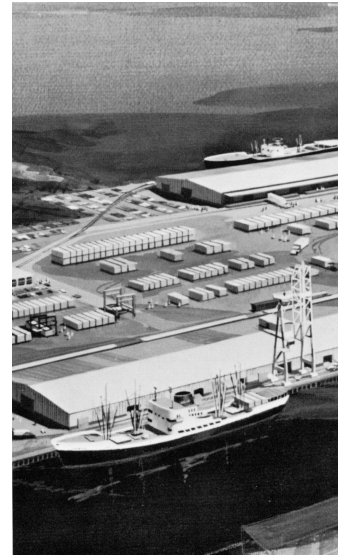
Figure 38 Drawing of Army Street terminal after its upgrade to containerization. Note that the ship at dock is t drawn as a hybrid breakbulk-container ship Source: Port of San Francisco Ocean Shipping Handbook 1966.
