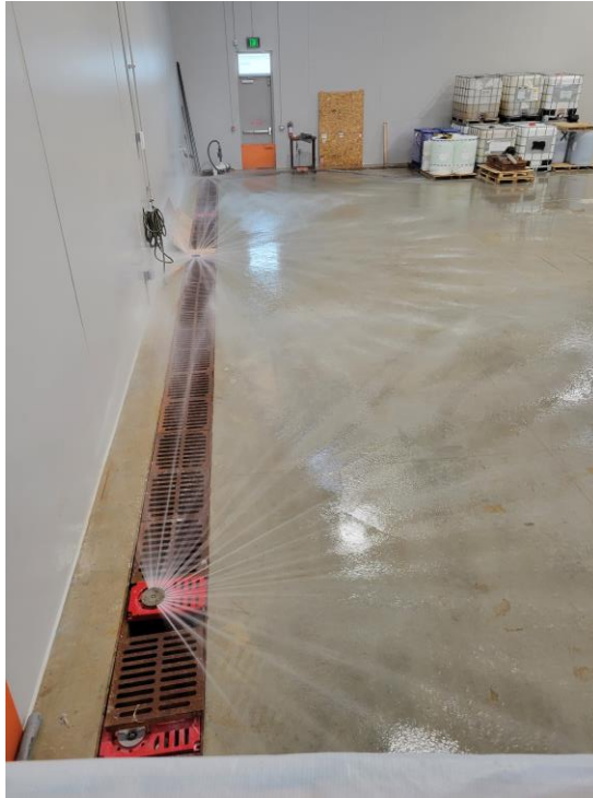
Figure 4-10. Viking Grate Nozzle 180° in reality
