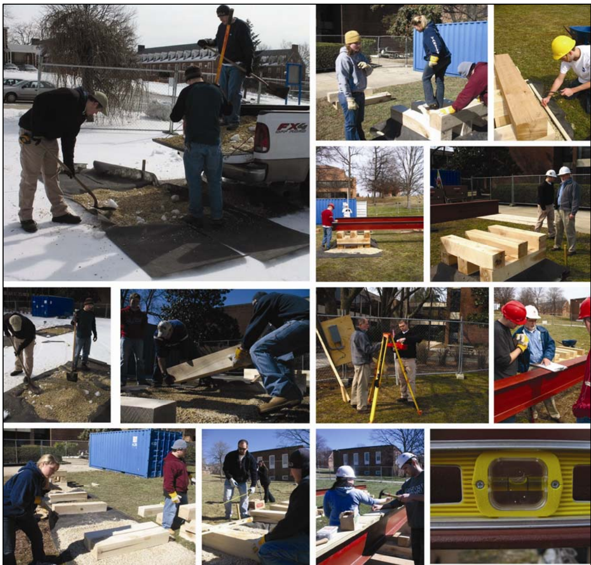
Figure 84: Foundation Sequence.
