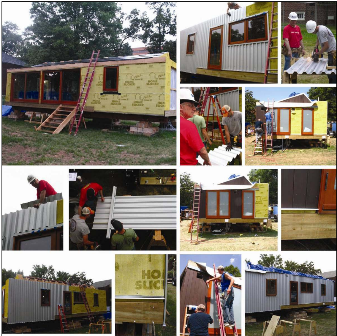
Figure 92: Siding Installation.
