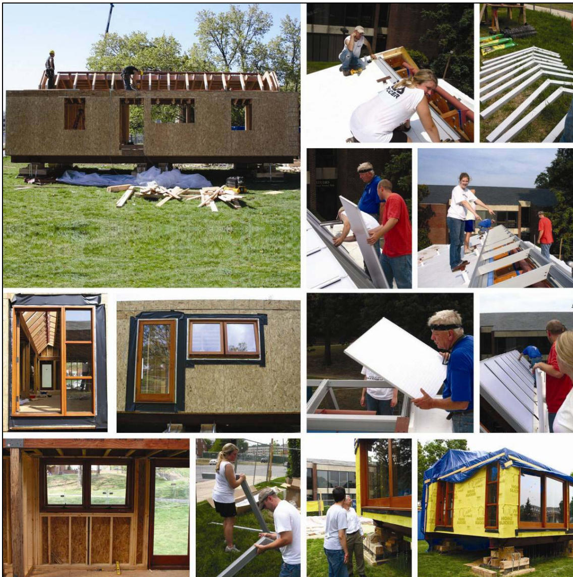
Figure 90: Door and Window Installation.
