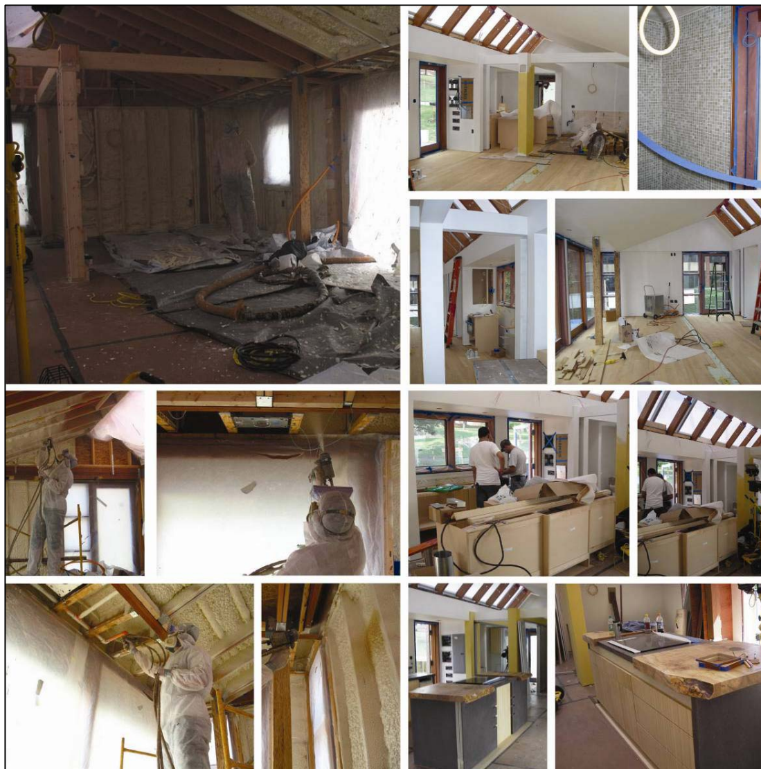
Figure 98: Insulation and Finishes Installation.
