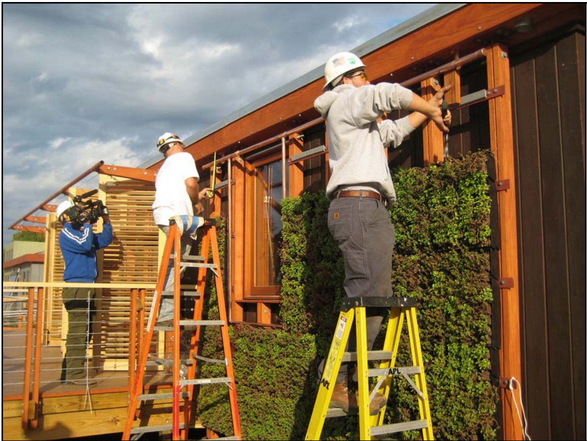
Figure 107: Installation of the Rainwater Filtration System
