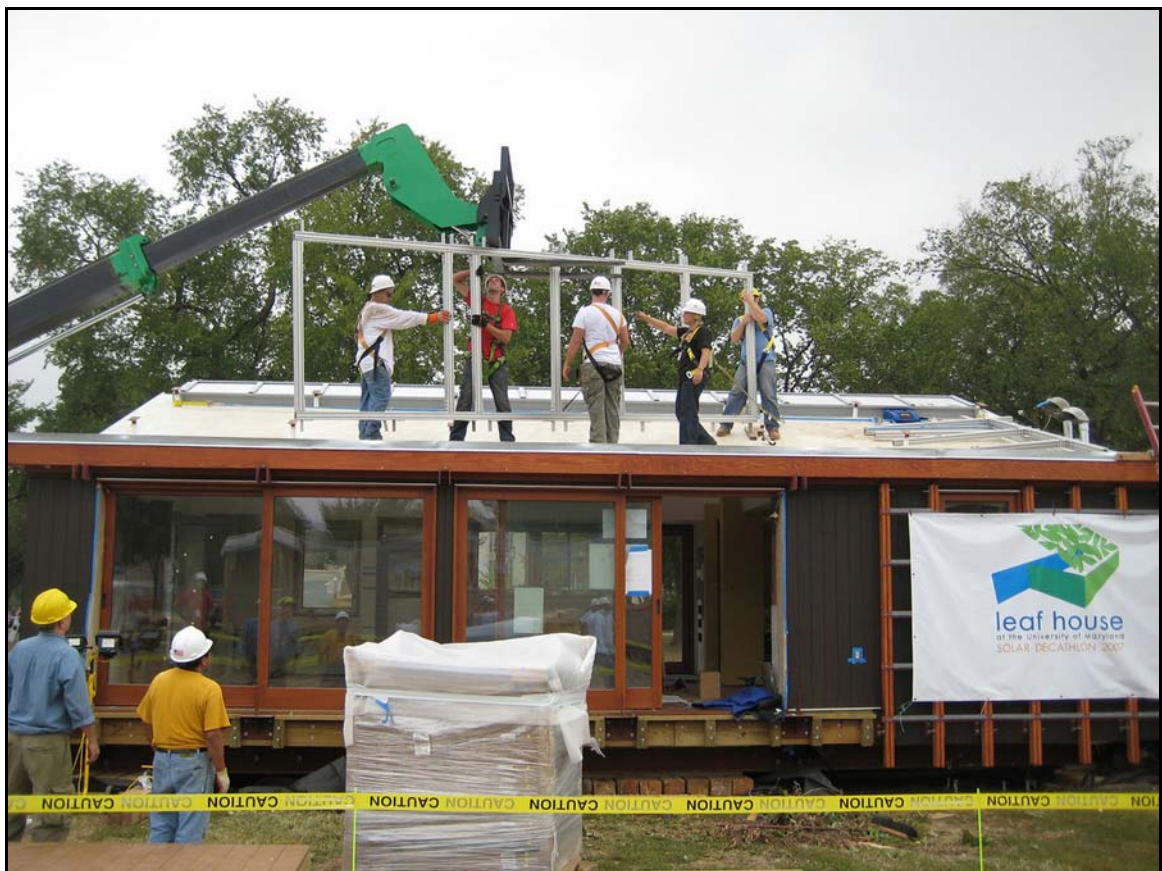
Figure 106: Reassembly of the PV Racking System
