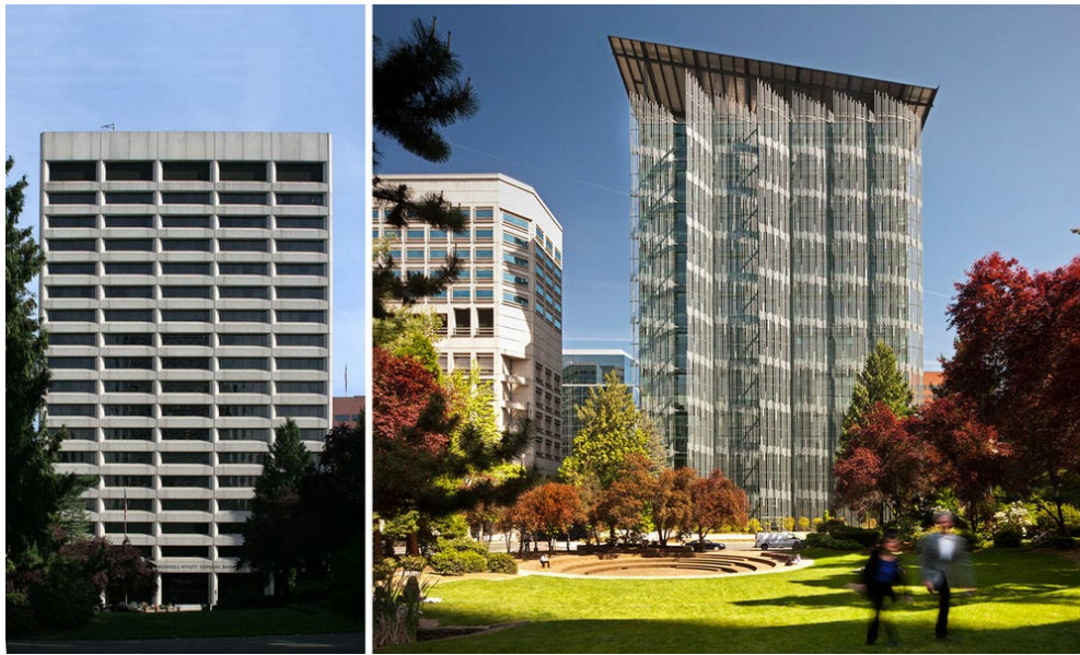
Figure 10 - Edith Green-Wendell Wyatt building before and after renovation images Source: https://www.aiatopten.org/node/354
