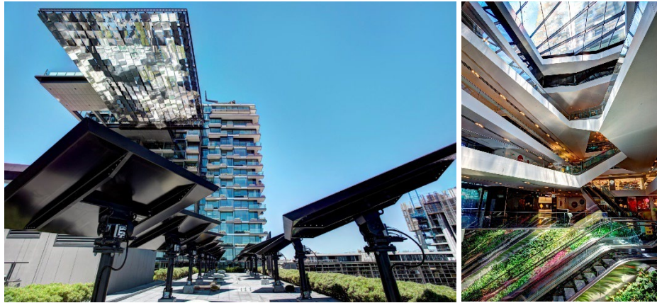
Figure 8 - Heliostat kinetic mirror system and naturally lit atrium space Source: https://good-design.org/projects/one-central-park-heliostat-and-reflector-system/
