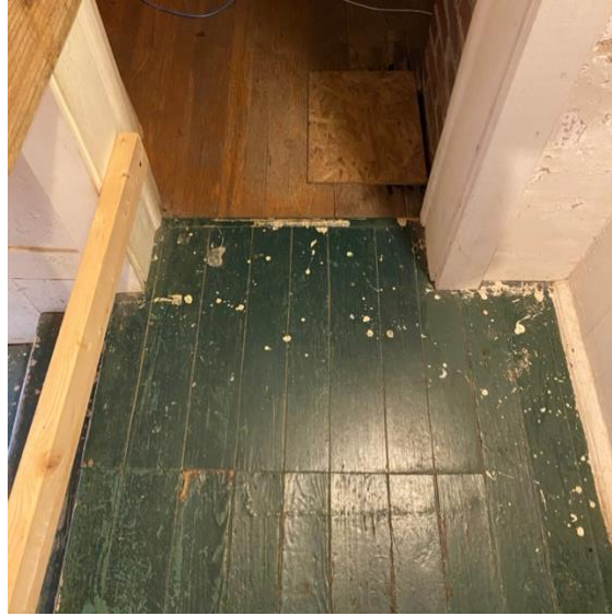
Figure 34. Ghost marks and infilled floorboards in Room 2E marking previous location of end chimney moved to exterior, staircase to first story at left ( Grant Cunningham, 2022 ).
