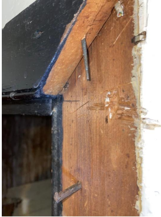
Figure 22. Machine-cut nails, door surround, Room 2D ( Grant Cunningham, 2022 ).
