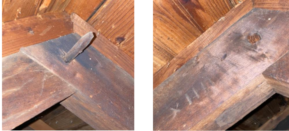
Figure 15. Phase I attic rafters showing pegged bridle joints and marriage marks ( Grant Cunningham, 2022 ).
