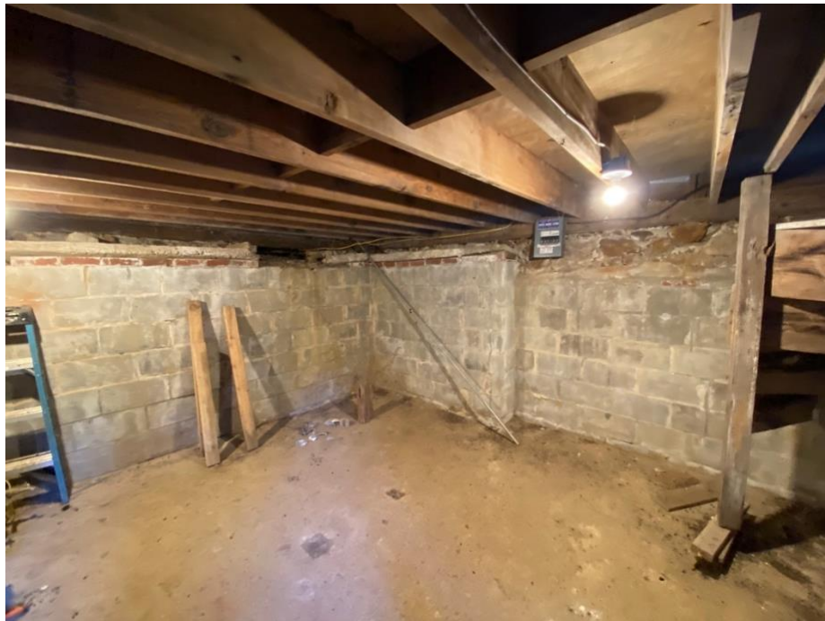
Figure 38. Cellar under Phase II (Room 0D) showing CMU walls, south and east elevations ( Grant Cunningham, 2022 ).
