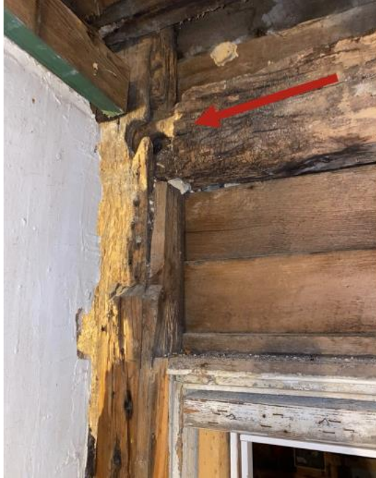
Figure 18. Overlapping notching near central passage partition wall ( Grant Cunningham, 2022 ).
