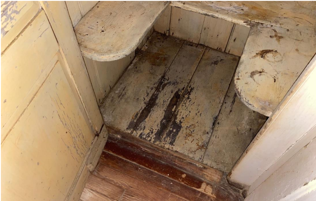
Figure 25. Original Phase I floorboards in staircase closet in Room 1B, newer floorboards at bottom ( Grant Cunningham, 2022 ).
