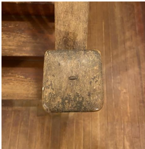
Figure 19. T-head wrought nails in central passage staircase newel post ( Grant Cunningham, 2022 ).
