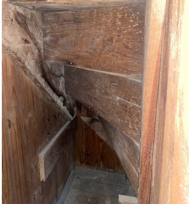
Figure 36. Circular sawn risers and machine-cut nails underneath attic staircase in Room 2D ( Grant Cunningham, 2022 ).
