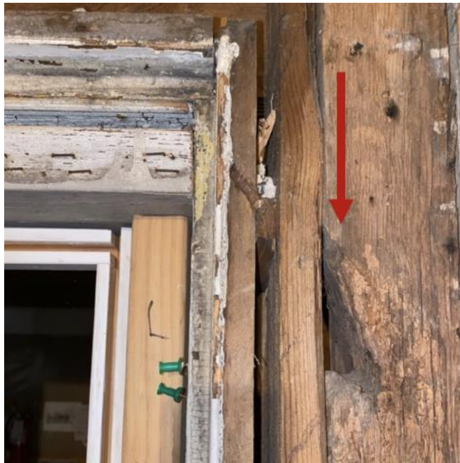
Figure 16. Notching for original entry door header, central passage ( Grant Cunningham, 2022 ).
