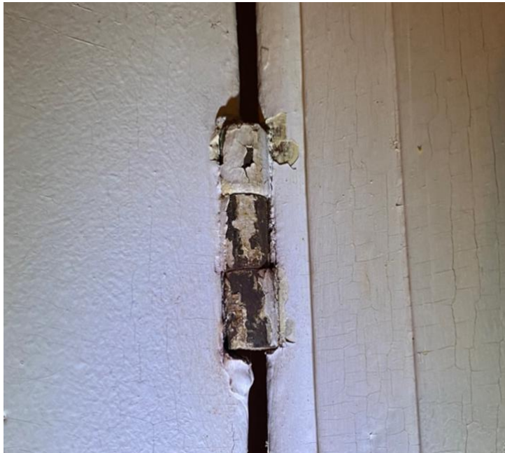
Figure 24. Mid-nineteenth century butt hinge on closet door in Room 2A ( Grant Cunningham, 2022 ).
