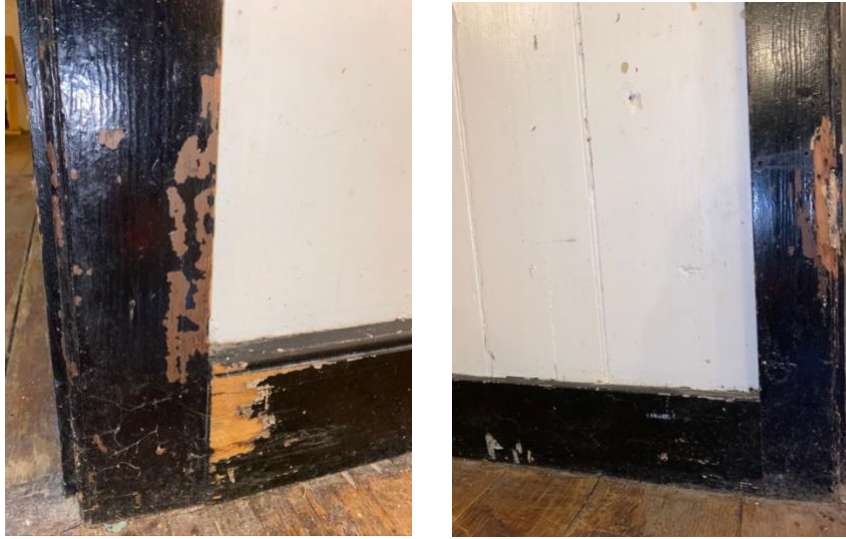
Figure 26. Original beaded baseboard (left) and replacement baseboard (right) in Room 2C ( Grant Cunningham, 2022 ).
