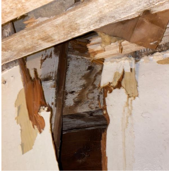
Figure 23. Whitewashed framing member visible under wall paneling ( Grant Cunningham, 2022 ).
