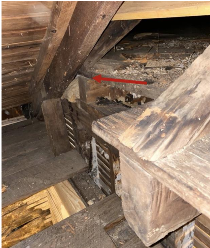
Figure 33. Phase I rafter end cut at joining of Phase II roof ( Grant Cunningham, 2022 ).
