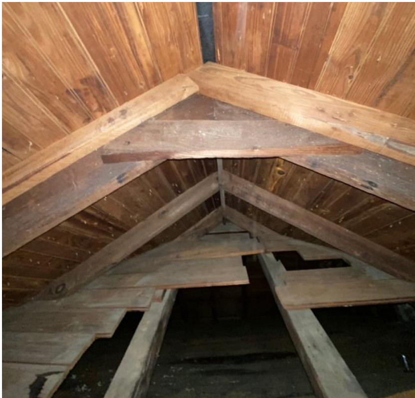
Figure 30. Original Phase II rafters joined without ridge board, foreground; later rafters joined at ridge board in Phase II roof extension, background; Phase One roof in far back ( Grant Cunningham, 2022 ).
