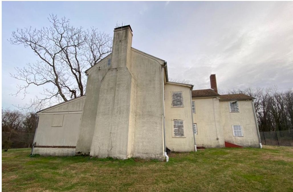
Figure 46. Goshen Farm House viewed from north, showing enclosed porch at left, stucco on all exterior elevations, and current building form with all phases visible ( Grant Cunningham, 2022 ).
