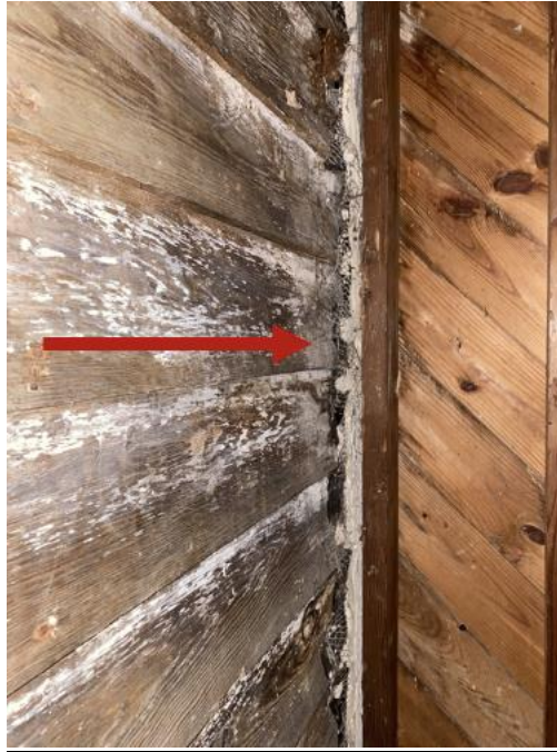
Figure 40. Remnants of stucco on the interior of the Phase III bathroom space, (Grant Cunningham, 2022).
