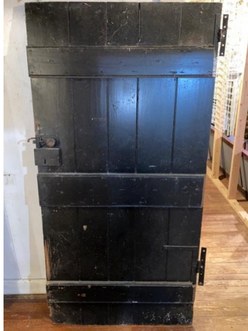
Figure 21. Board-and batten-door separating Room 1A and Room 1B (hall and central passage) featuring HL hinges and handmade screws ( Grant Cunningham, 2020 ).
