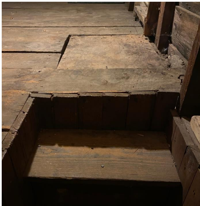
Figure 37. Attic staircase in Room 3B, showing floor patch where interior end chimney was previously located ( Grant Cunningham, 2022 ).
