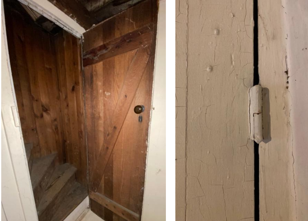
Figure 35. Second-story staircase to attic in Room 2D, featuring a board and batten door at bottom with cut nails ( Grant Cunningham, 2022 ).
