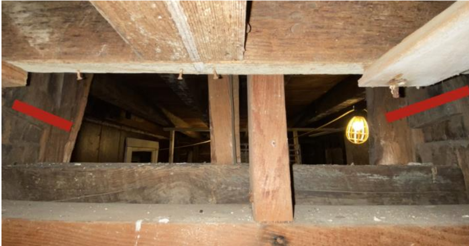
Figure 27. Notching for window header above doorway from Room 1C to Room 1D (Grant Cunningham, 2022).
