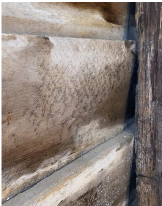
Figure 14. Circular sawn weatherboard siding in Phase I house ( Grant Cunningham, 2022 ).
