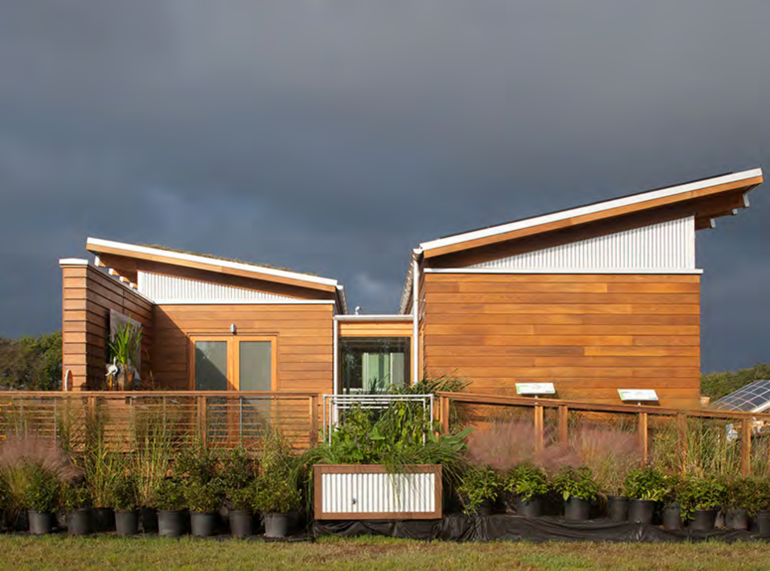
University of Maryland's WaterShed, 2011 Solar Decathlon Entry
