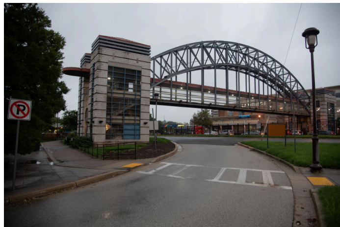
Fig 53. Pedestrian footbridge over MD-410 (East-West Highway) in Hyattsville.
