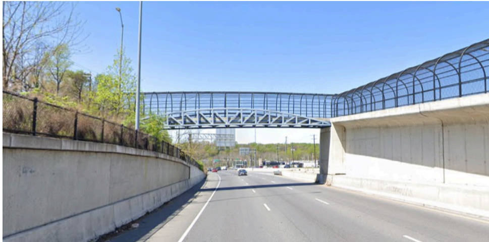
Fig 54. Pedestrian Bridge over MD-5 Southbound in Camp Springs.
