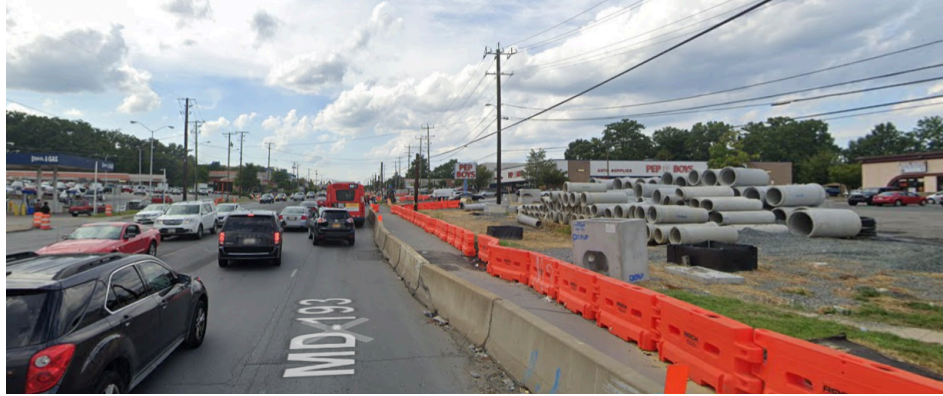
Fig 57. There is a gap in the sidewalk on the north side of University Blvd to the west of the Riggs Road intersection.
