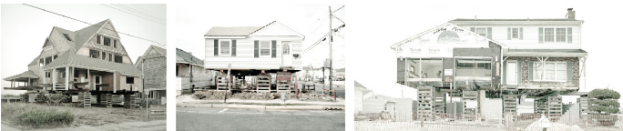
New Jersey house raising, Ira Wagner
