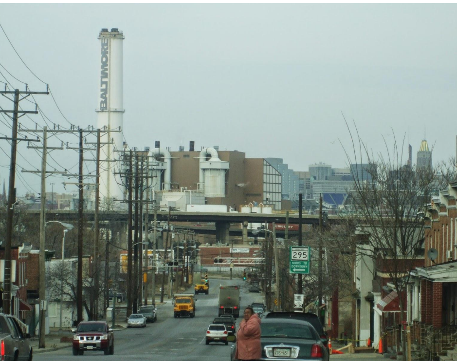
WESTPORT: ANNAPOLIS RD + INCINERATOR
