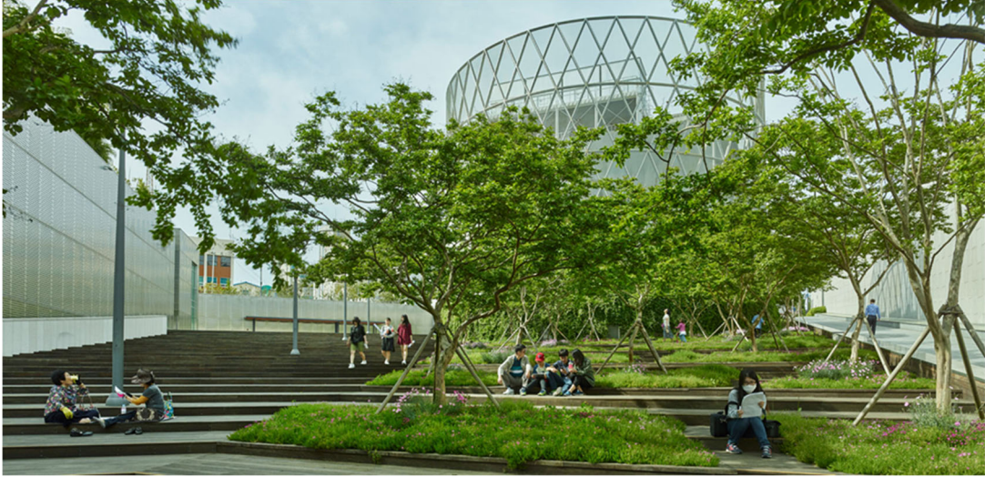
Figure 33, The Asia Culture Center in Gwangju, South Korea, (Kyu Sung Woo Architects)
