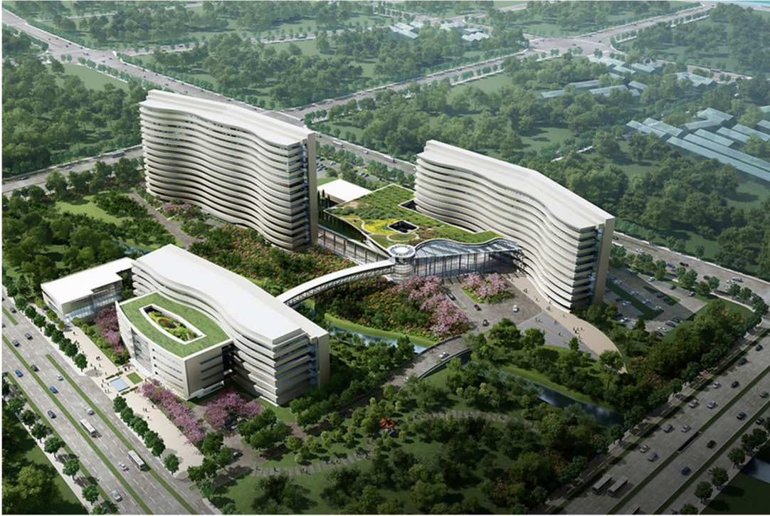
Figure 27, Wuxi Women's and Children's Hospital, (Perkins Eastman)
