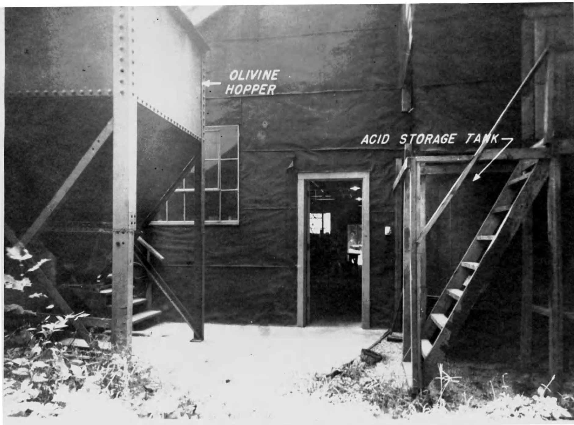
Fig. 8— Raw Material Storage
