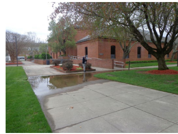
Figure 2.42 Eastern view of EFPAC Building.
