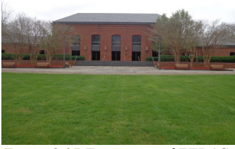
Figure 2.37 Front view of EFPAC Building.
