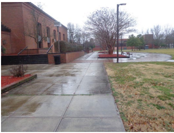
Figure 2.40 Western view of EFPAC Building.
