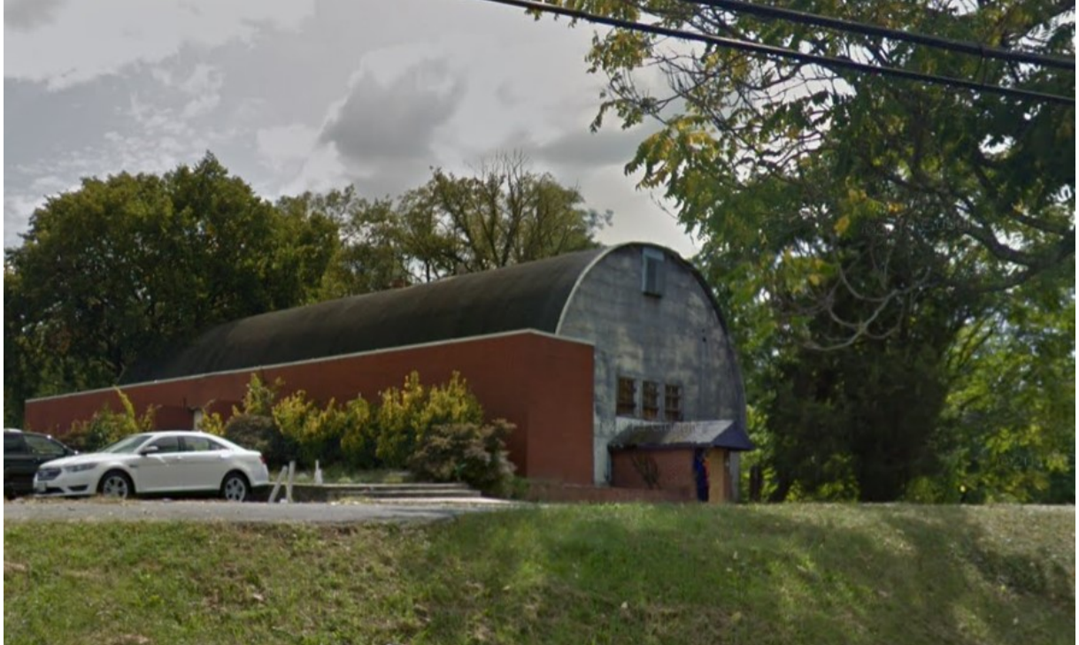
Figure 45. Northwest elevation of the Quonset Inn in 2017. Source: Google, 2017.
