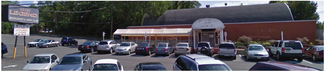
Figure 43. North Elevation of the Quonset Inn in 2009. Source: Google, 2009.
