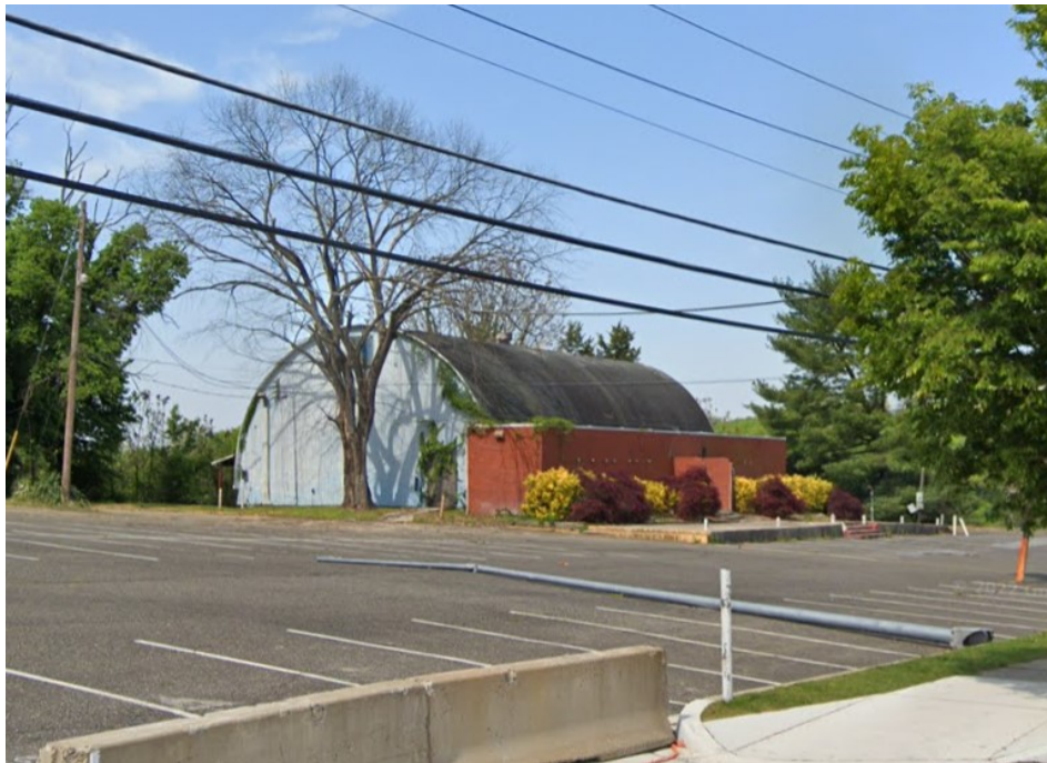
Figure 46. Northeast Elevation of the Quonset Inn, 2022. Source: Google, 2022.
