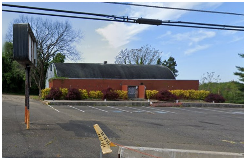
Figure 42. North Elevation of the Quonset Inn in 2022. Source: Google, 2022.
