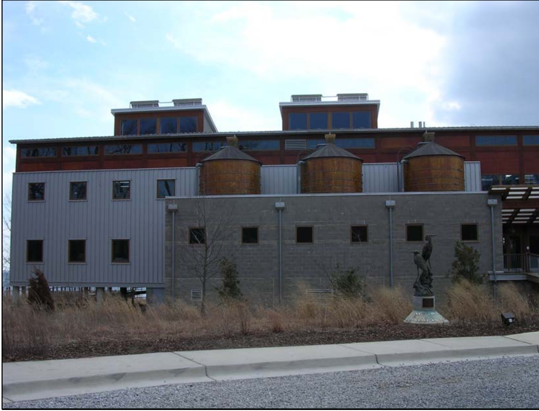
Figure 44 The building reuses rainwater captured off the roof in three large cisterns.
