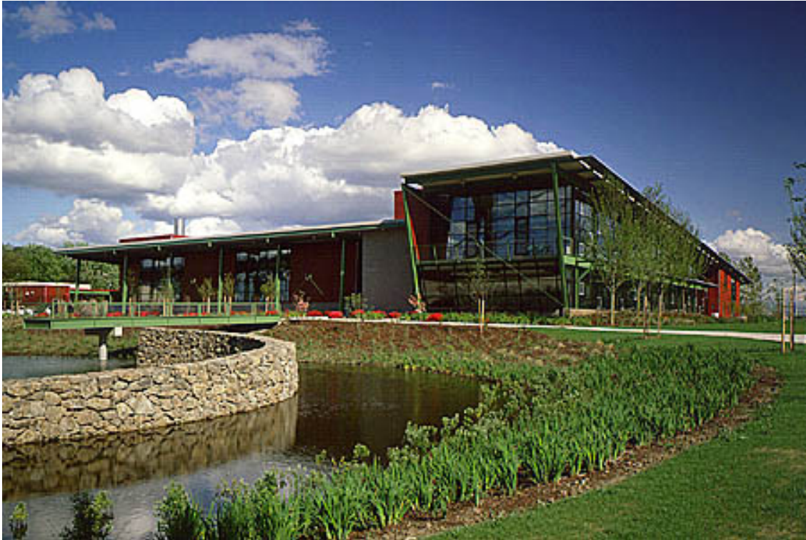
Figure 46 Demonstration Water Treatment Ponds. Rain on the roof is routed into this pond. The process of storm water treatment became clearly visible to public. 12
