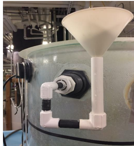
Figure 4.2 Additions port with funnel on side of reservoir tank. Piping filled with deionized water.
