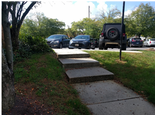
(a) Wheel-chaired inaccessible (Staircase on a sidewalk).
