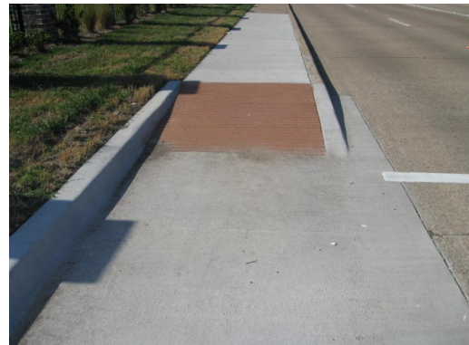
(b) Wheel-chaired accessible (Ramp on a sidewalk).
