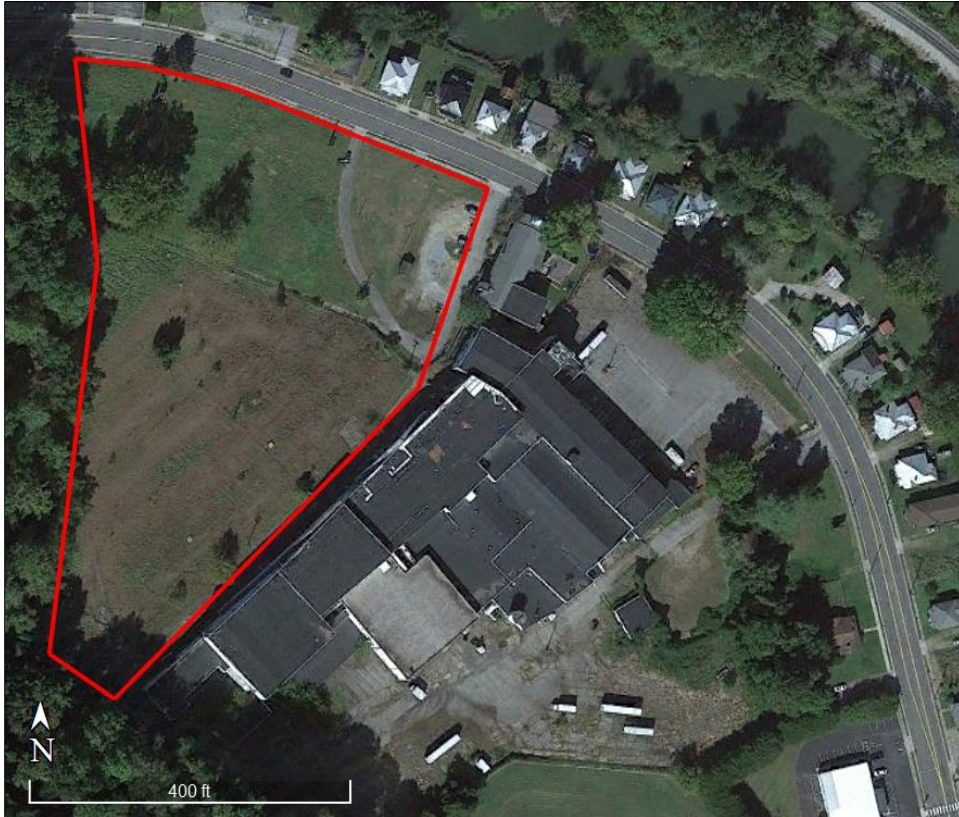
Figure 16: Aerial view of the project area, showing factory immediately east and extant workers housing across Fairystone Park Highway from the project area. Source: Google Earth 2021, graphic by the author.
