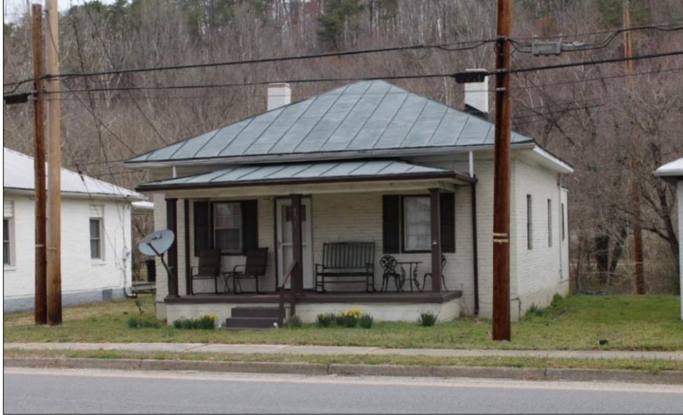
Figure 8: Worker housing near 44HR0219, VDHR #044-5180-0018. This and neighboring dwellings retain much of their historic character described by Blanton et al. 2009. Courtesy of D+A (2021:7-16).
