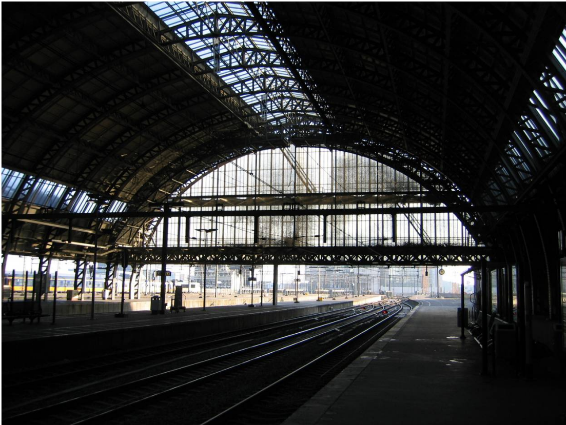
Figure 130 - View of Existing Train Shed
