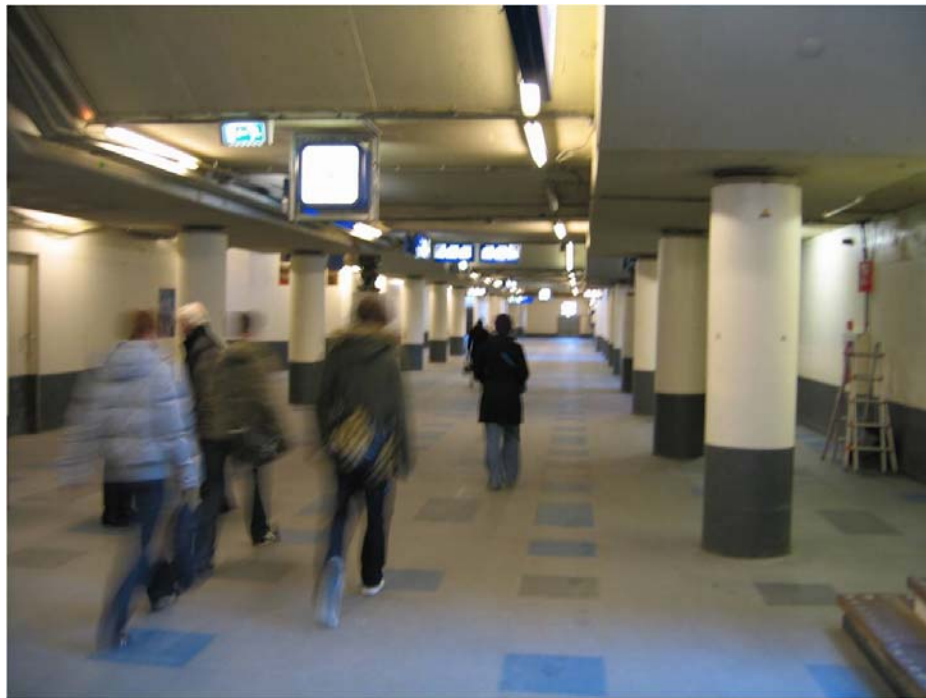
Figure 67 - Existing Central Passage
