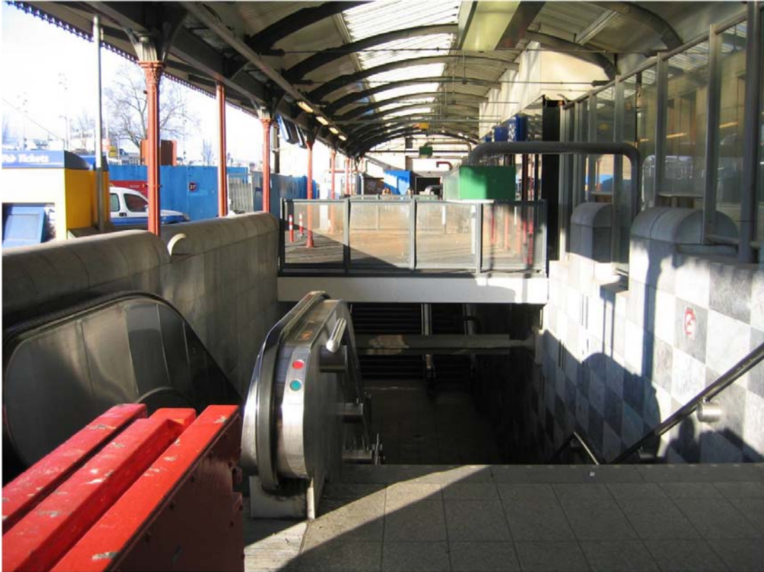
Figure 162 - Before: Metro Entrance
