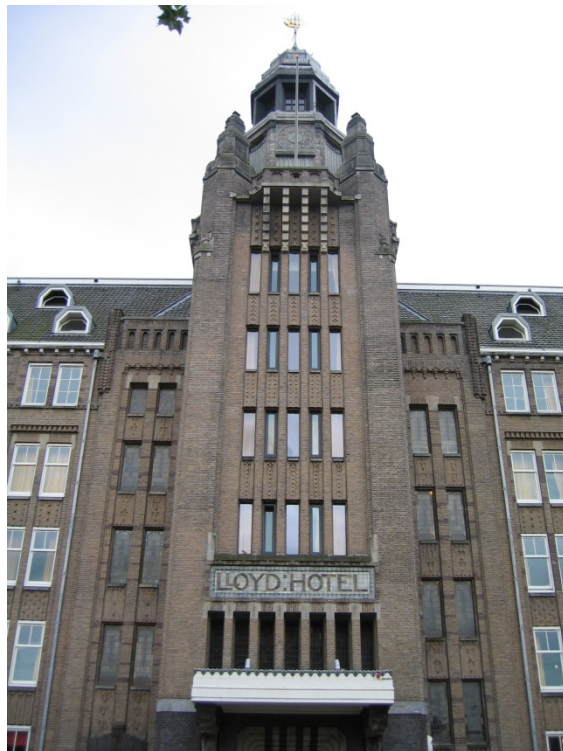
Figure 7 - Lloyd Hotel / Brick Detailing
