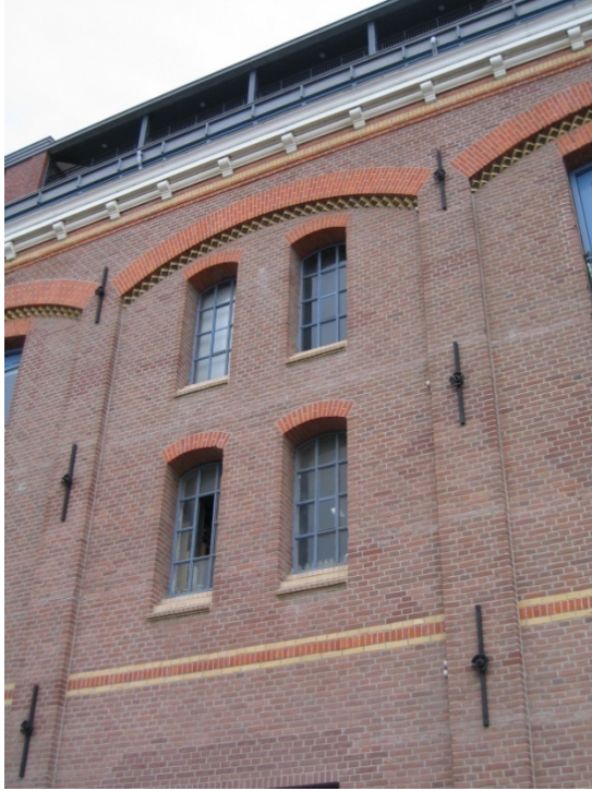
Figure 6 - Old Waterfront Warehouse / Brick Detailing
