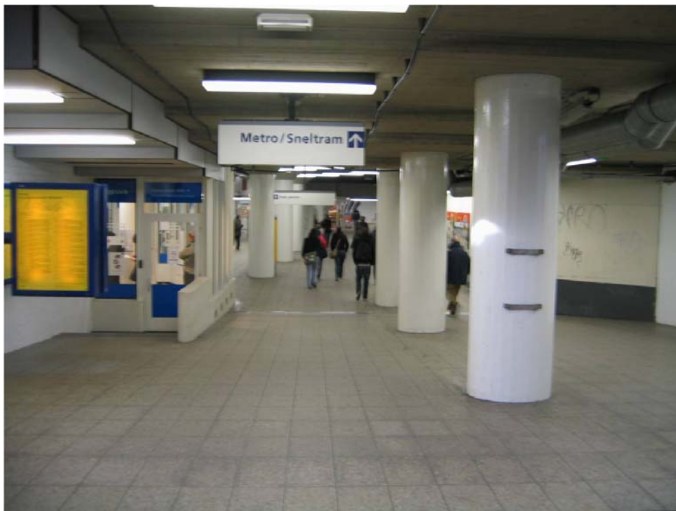
Figure 111 - View of Existing Metro Station
