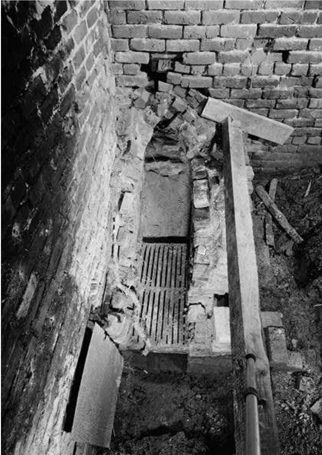
Figure 9 - Hypocaust furnace – Picture taken of the Wye Greenhouse furnace prior to its complete destruction. Photo circa 1963 for the Historic American Buildings Survey (HABS).
