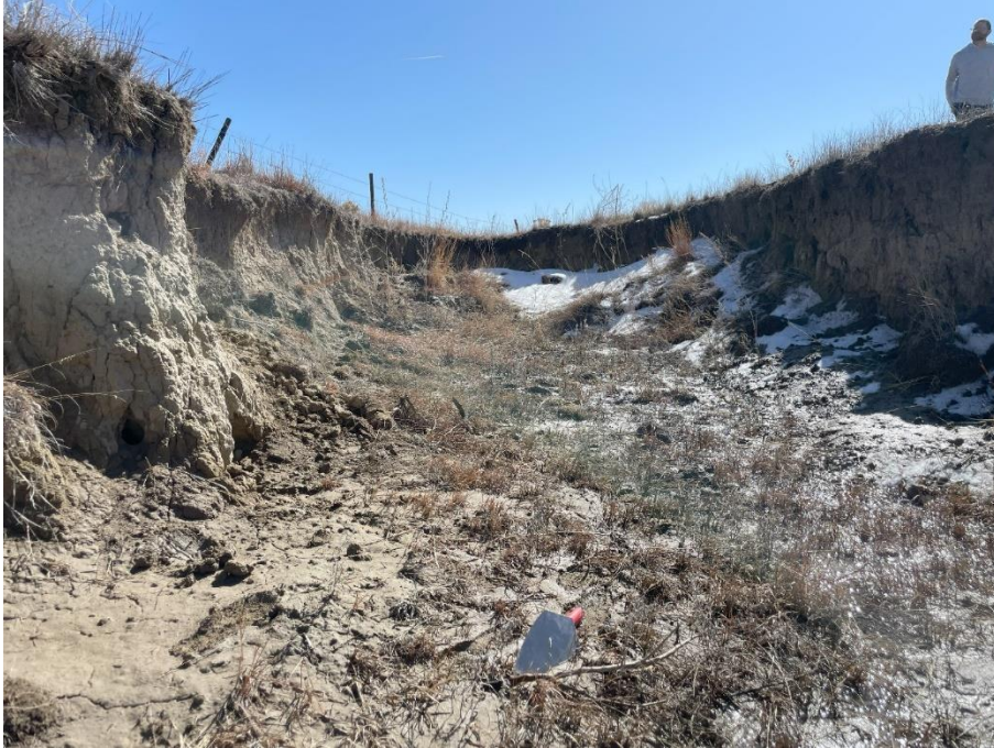
Figure 5.15. Ground view of the end of Site #1. Photo taken by author.
