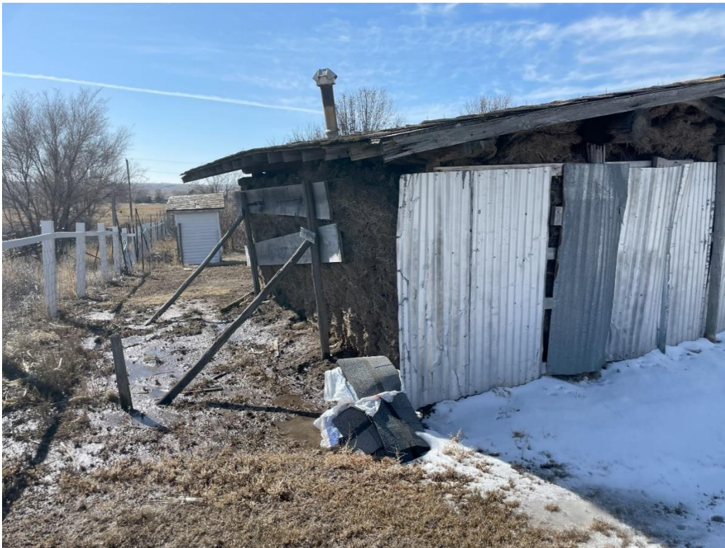
Figure 5.21. Perks family Sod Home wall reinforcements, taken by author.
